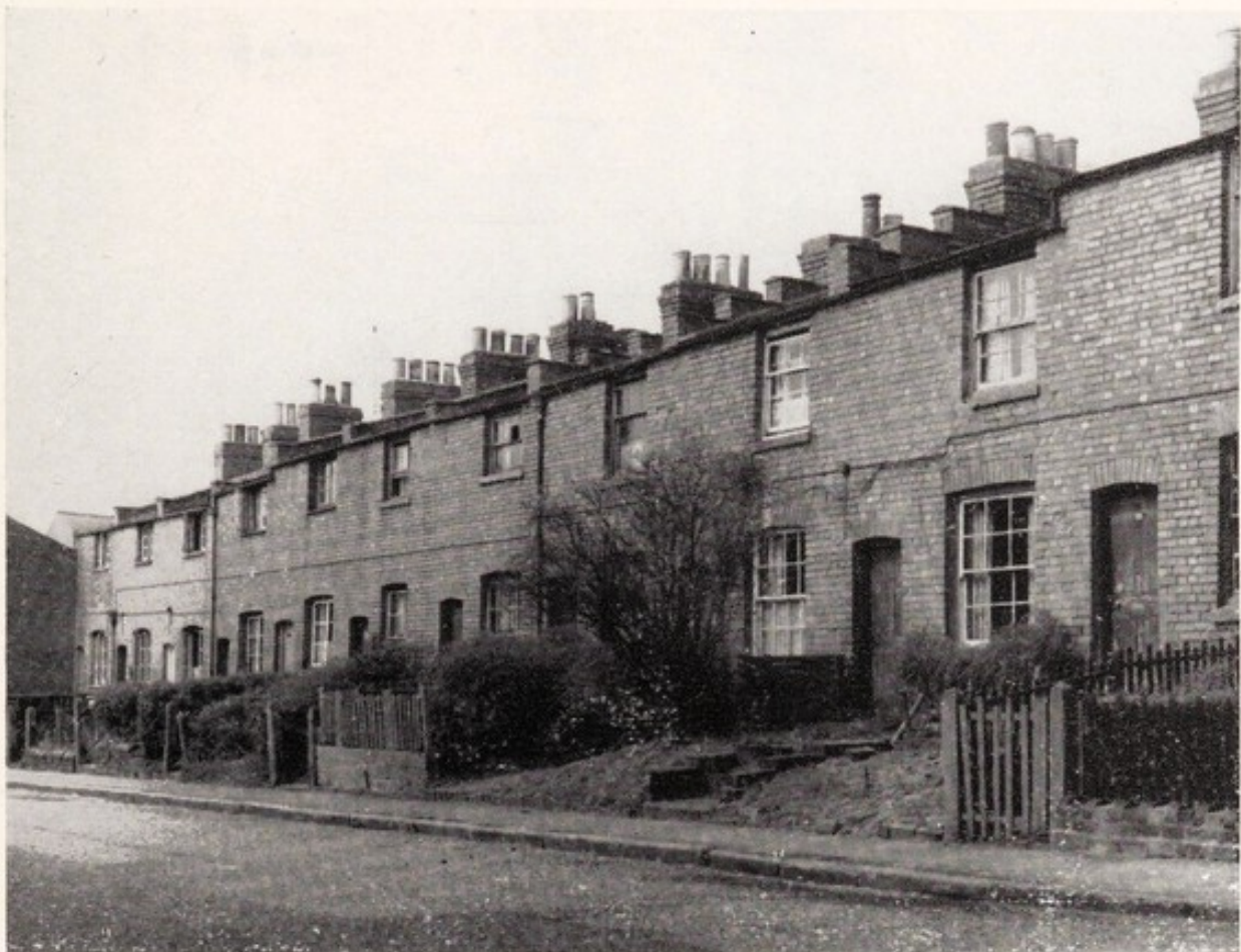
HAMPTON STREET (NORTH SIDE).
