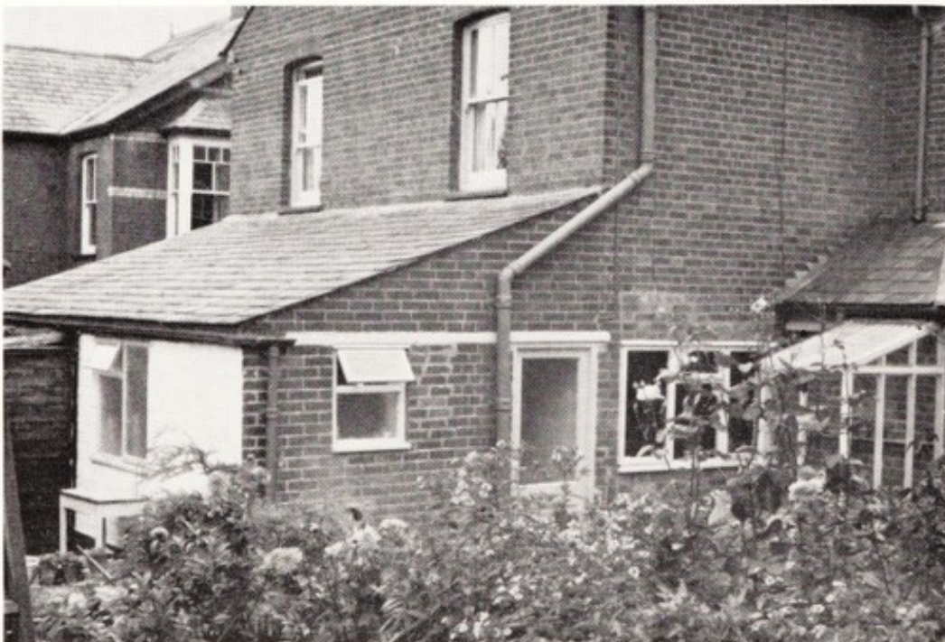
Provision of modern kitchen and bathroom with separate internal W.C. in semi-detached house built 1900. Rear door, moved to new intervening lobby, obtains better arrangement of kitchen and work sequence, and allows for larger window.
