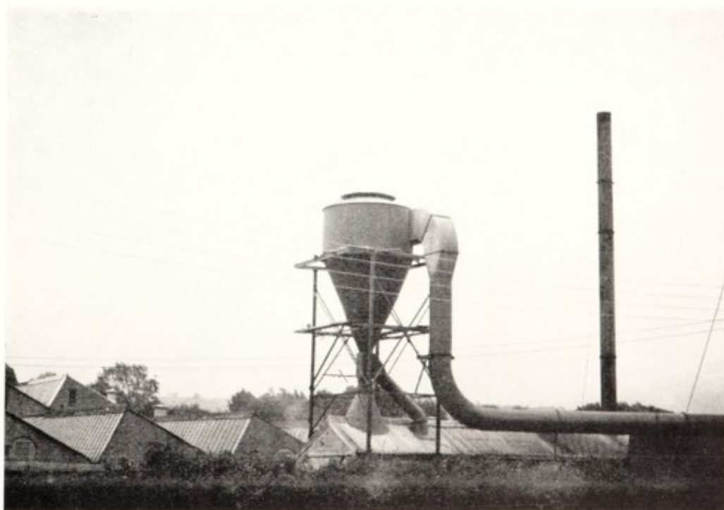
Modernisation of Plant. Installation of special feeder mechanism to utilise factory wood waste as main fuel.
