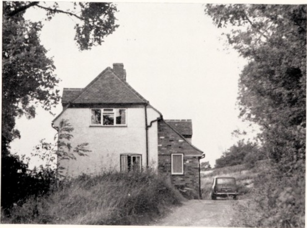
Repair and improvement of an unfit cottage.
