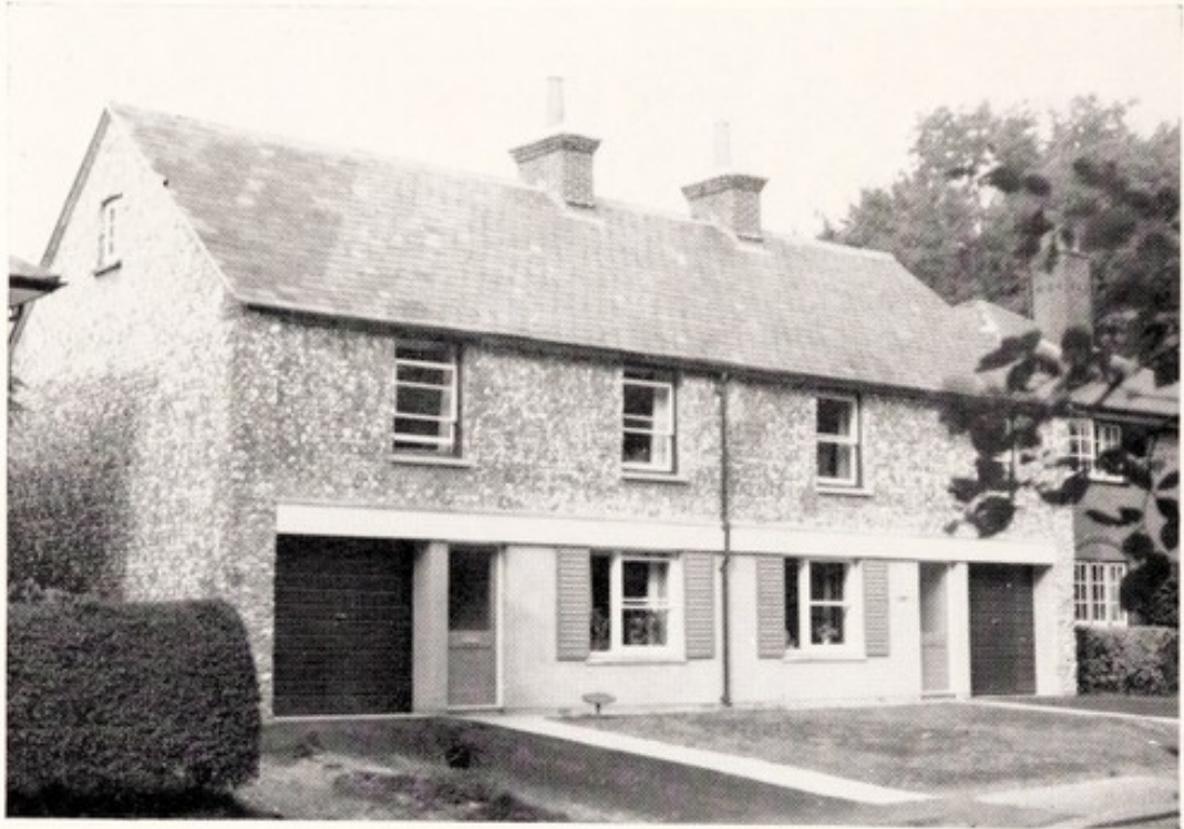
Four unfit cottages converted, repaired and improved to form two three-bedroom houses, with integral garage.
