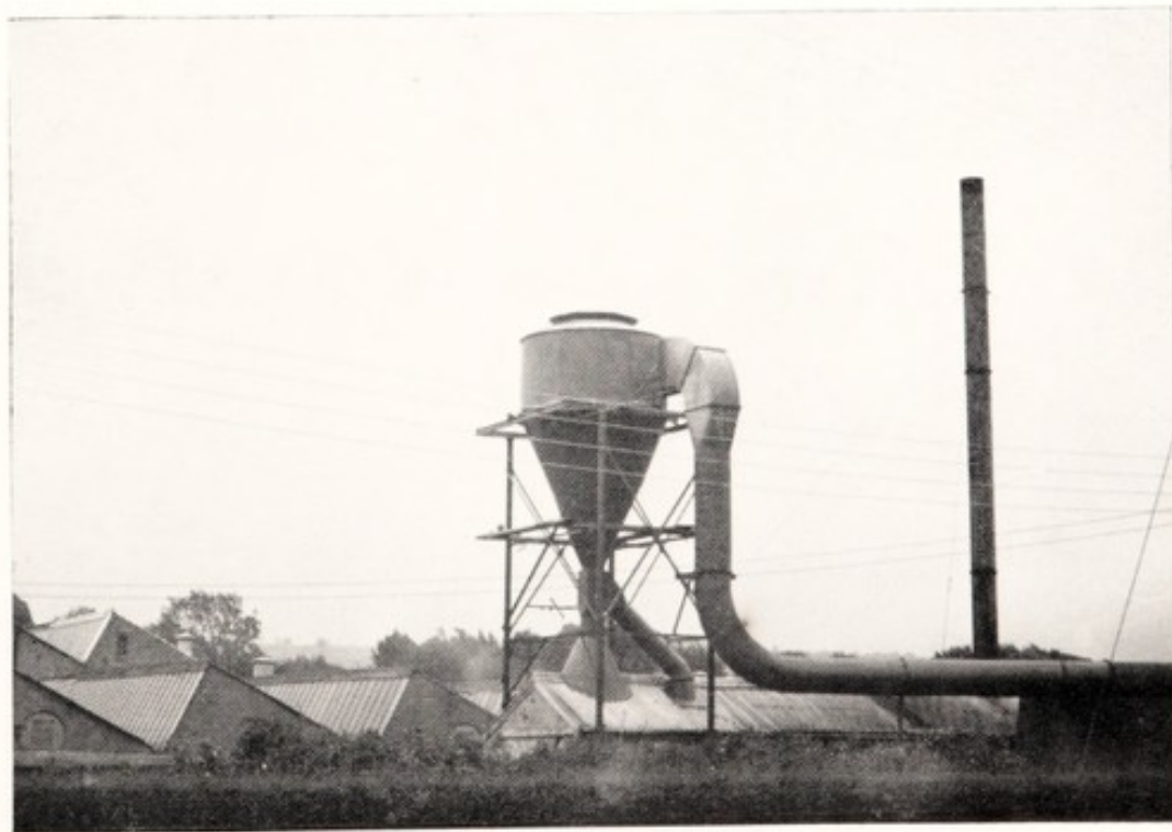
Modernisation of Plant – utilising factory wood waste as main fuel
