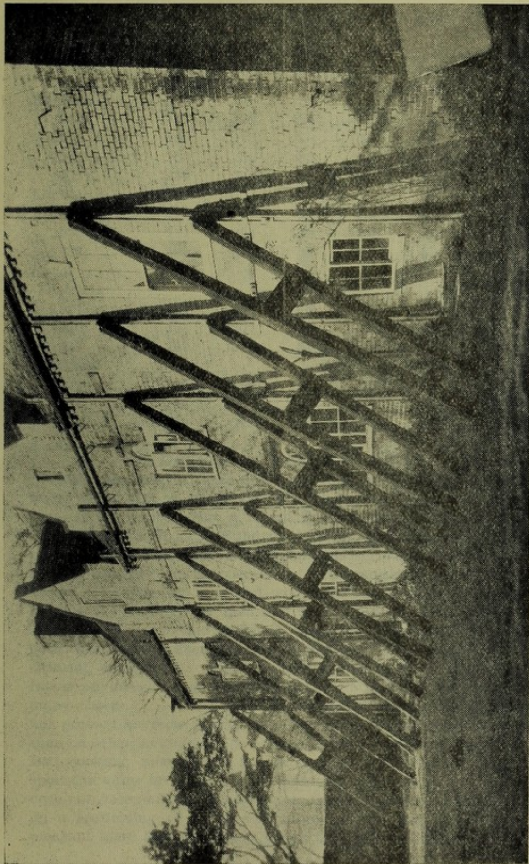
FIG 3.—Shoring of Building due to Ground Subsidence.
