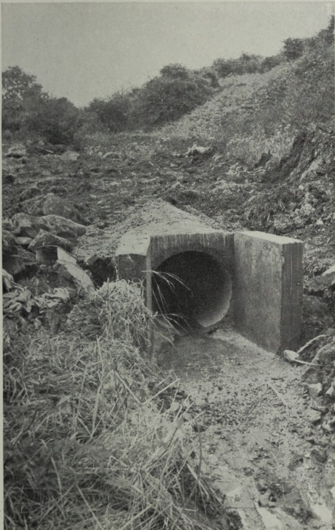
Oakdale Farm, Harrogate — showing culverting of stream prior to the valley being bridged by refuse; commenced May, 1968.
