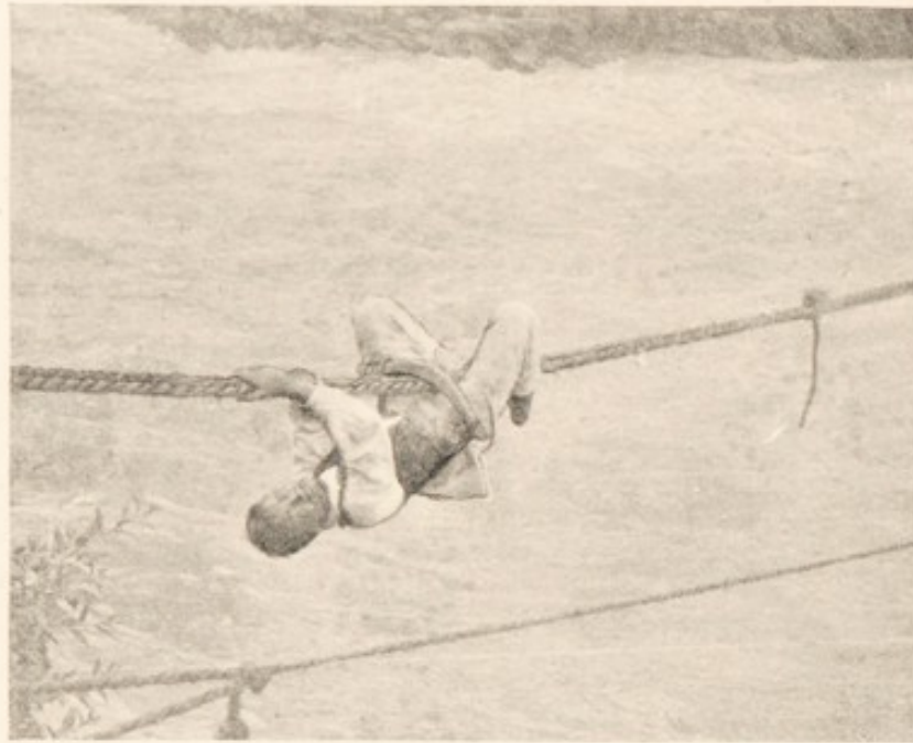
NATIVE CROSSING ROPE BRIDGE
