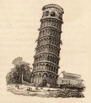
\* The dimensions of this tower contract as you ascend it, and the thickness of its walls is greatly less at the top than at the bottom. Both these causes have a tendency to bring its centre of gravity below the middle point in the height of the tower; and thus, the vertical through that point, further within the boundary of the base.
