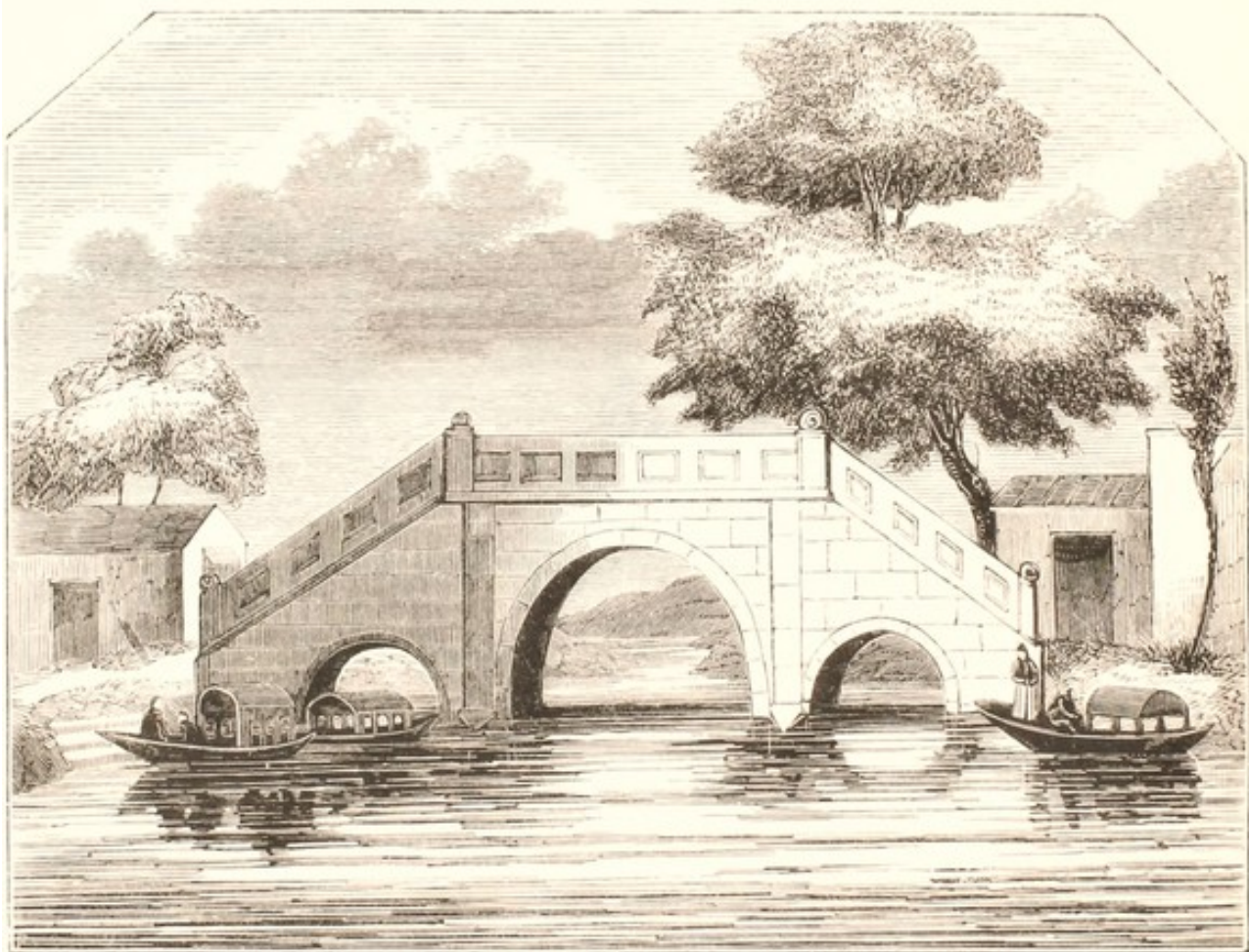
BRIDGE AT HONAN.
