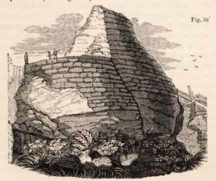
Shift or "fault" in the Round Tower of Terranuova in Calabria, occasioned by the earthquake of 1783.
