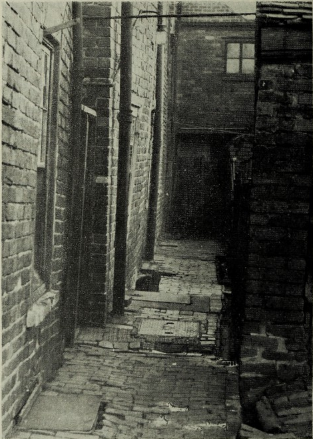
The rear walls of this property are badly bulged and twisted. Attention is also drawn to the congestion and the insanitary state of the paving.
