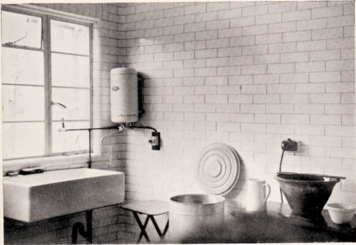
View of compartment adapted for use by producer of a COLD MIX. Note minimum requirements of glazed wall surfaces, adequate light and ventilation, glazed sink, hot-water geyser, boiler for sterilization and enamel topped table.
