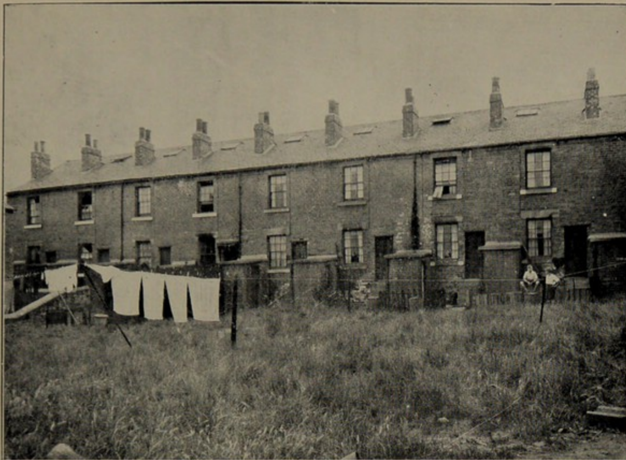
Fig. 10A— Sub standard houses, terraced row. Note sanitary conveniences at the rear of the dwelling. This type will have to be dealt with when the worst of the clearance areas are rehoused.
