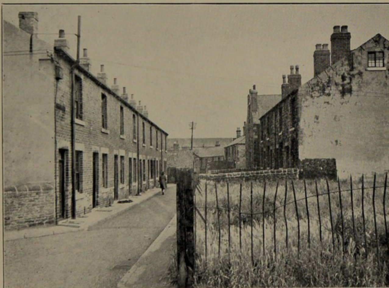
Fig. 10B— Front view of terraced row shown in Fig. 10A. Note the narrow front street congested siting.
