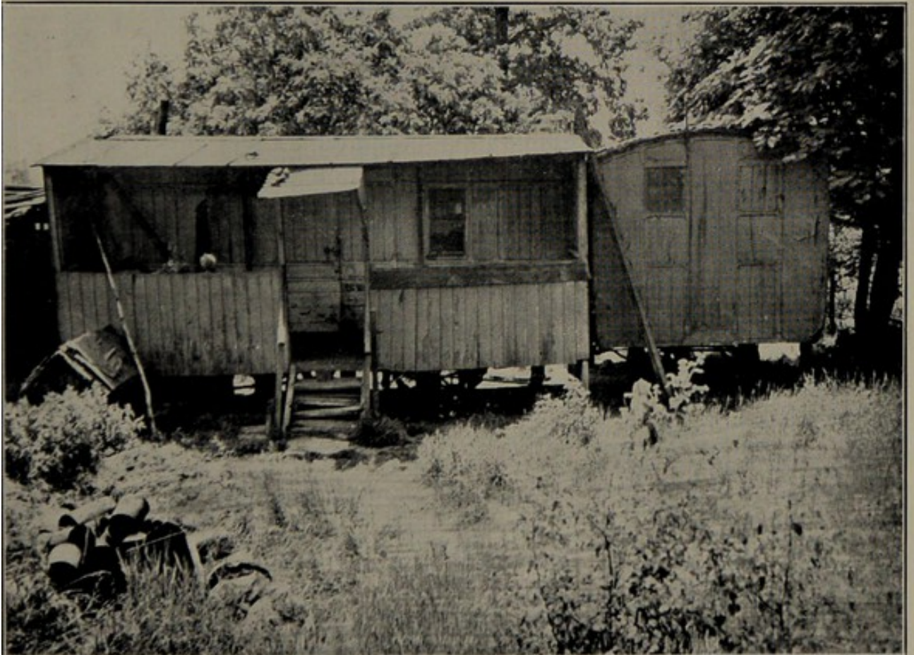
Fig. 4—Caravan Subject to Demolition Order.
