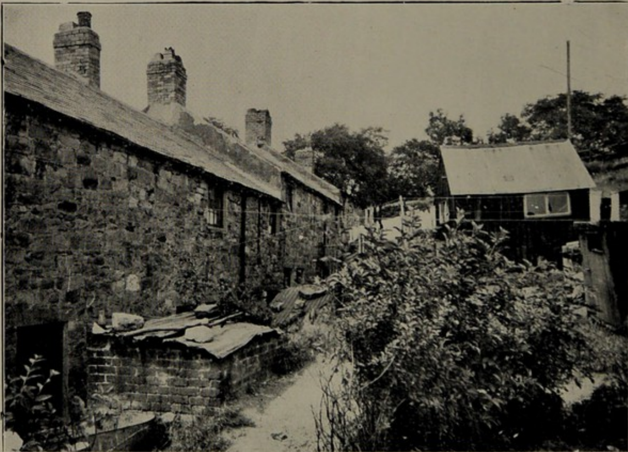
Fig. 2—Typical Clearance Area Property.
