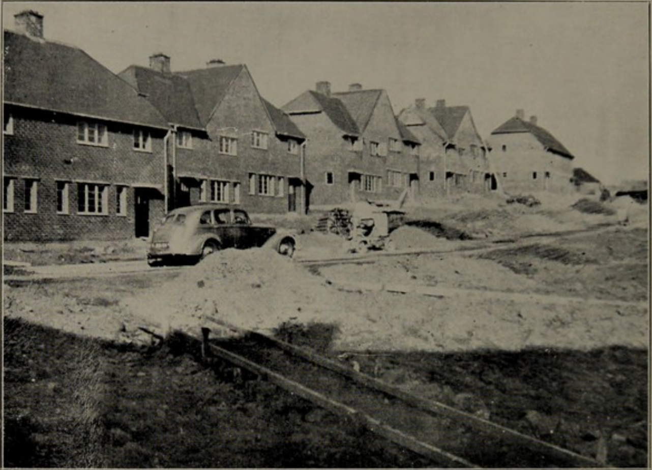
Fig. 5—Traditional brick houses under construction.
