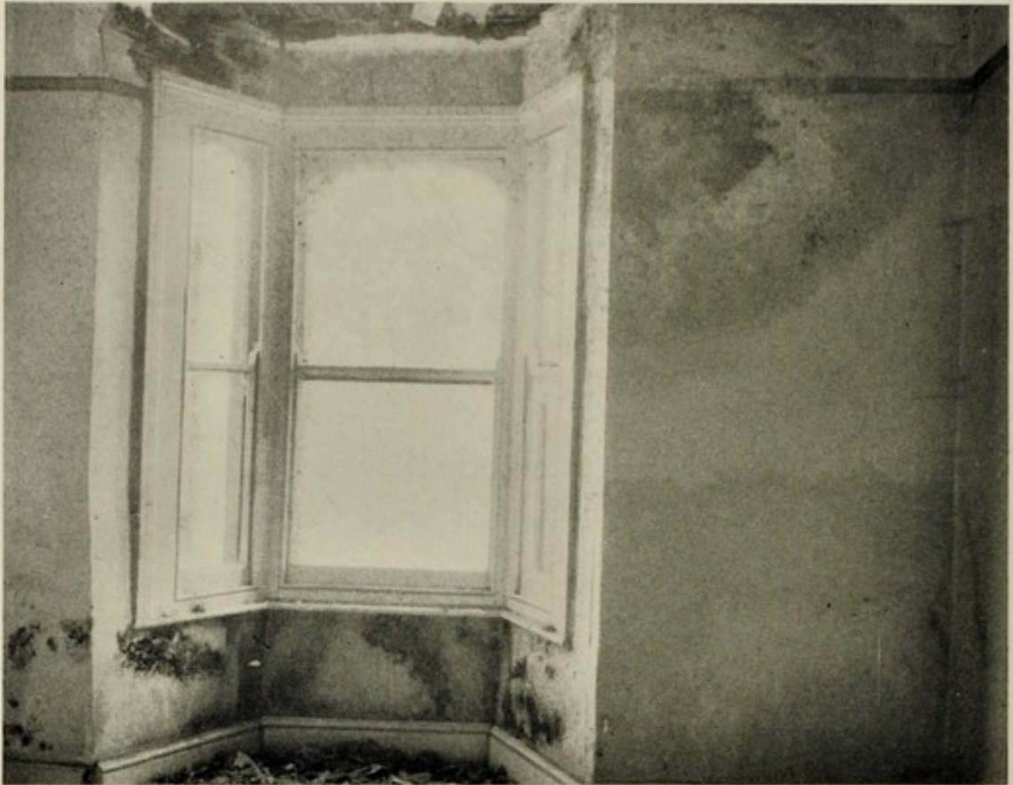
Front Living Room: The roof has collapsed under this old window, the joists are rotten and extensive areas of damp and defective plasterwork exist due to neglected deteriorations.
