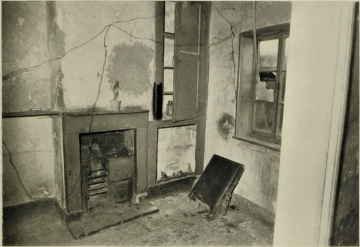
View of the kitchen from the entrance doorway, showing broken stone floor, defective grate, extensive disrepair and dirty and dilapidated conditions.
