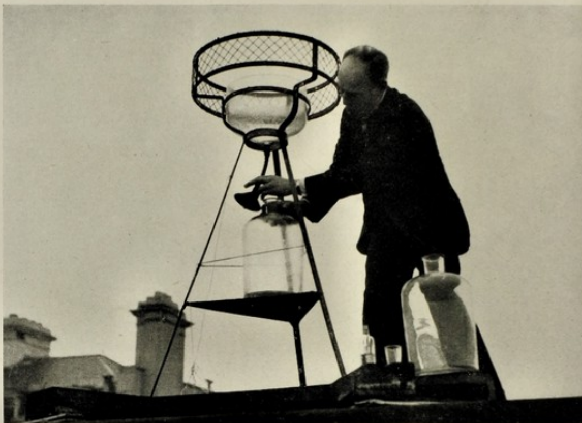
Smoke Abatement—Deposit Gauge in Action
