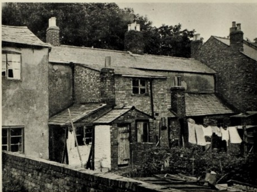
Rear view of three houses in block prior to reconditioning.
