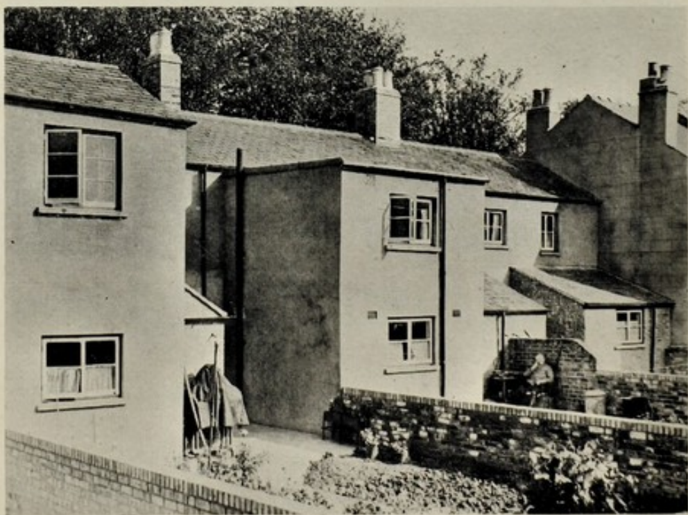
View of above houses on completion of work.
