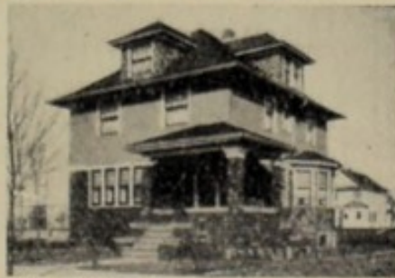
A No. 4121 IDEAL Boiler and 470 ft. of 34-in. AMERICAN Radiators, costing the owner $180, were used to heat this cottage. At this price the goods can be bought of any reputable, competent Fitter. This did not include cost of labor, pipe, valves, freight, etc., which installation is extra and varies according to climatic and other conditions.
