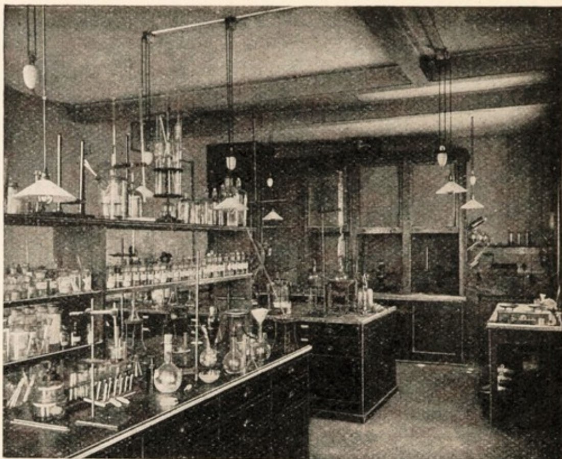
THE LABORATORIES, THIRD FLOOR
