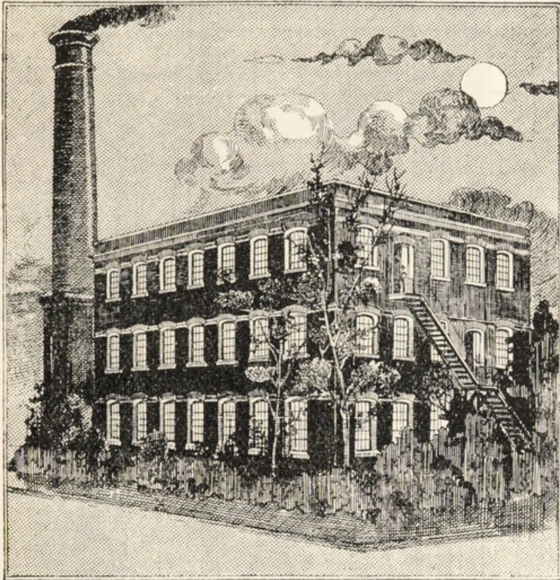
ADDITIONAL LABORATORIES recently completed at Burroughs Wellcome and Co.,'s Works at Dartford.
