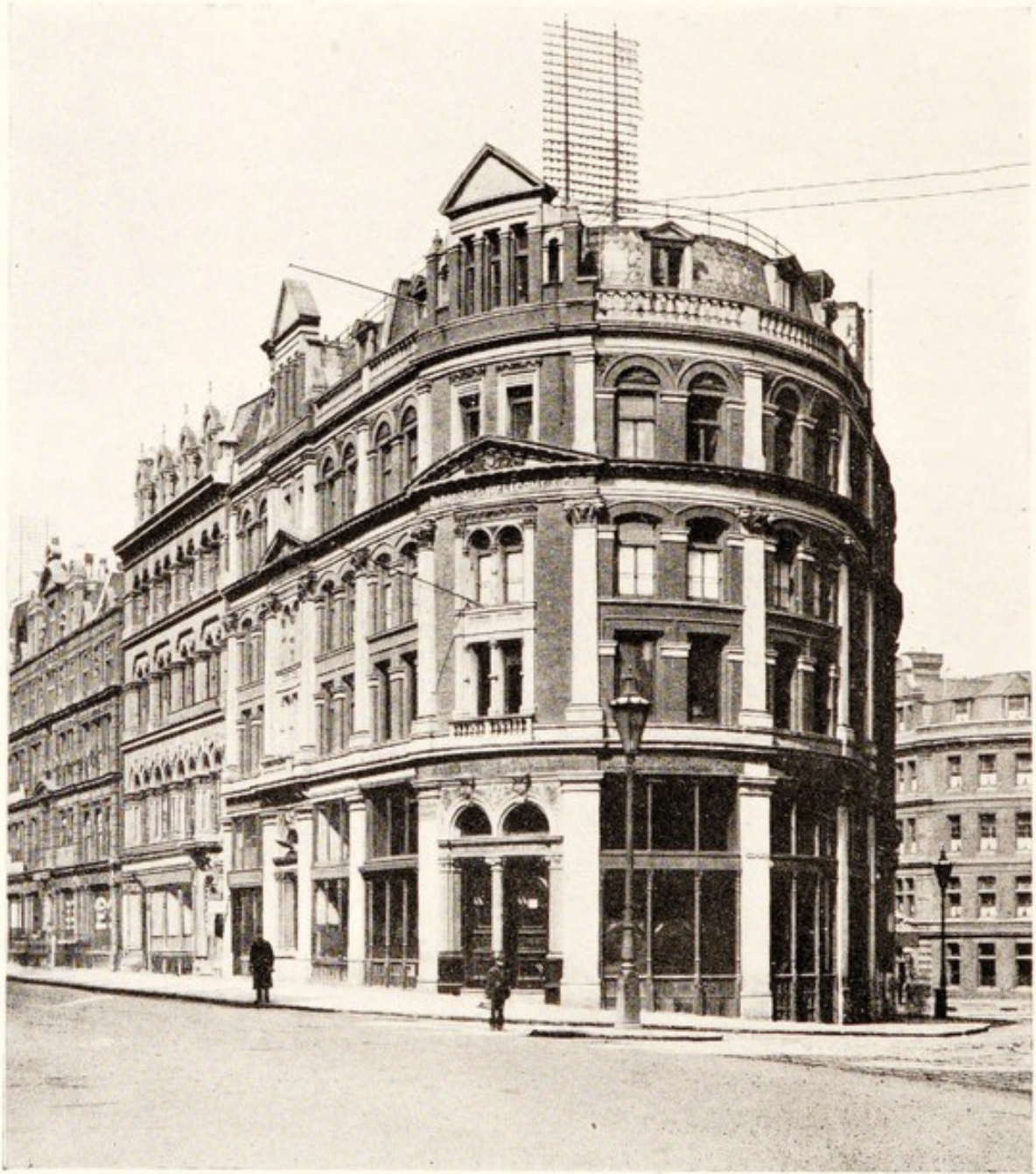
PORTION OF FRONTAGE BURROUGHS WELLCOME & CO.'S CHIEF OFFICES, LONDON Corner of Holborn Viaduct and Snow Hill facing Holborn Viaduct Station
