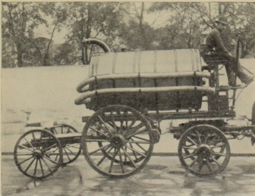
Fig. 30.—"Odorless excavator" tank wagon, with pump as a trailer.
