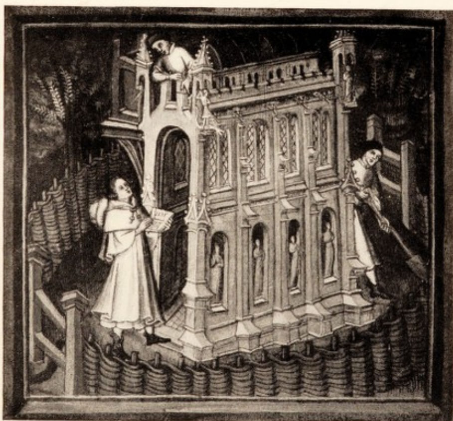
BUILDING THE CHAPEL ST. FREMUND
