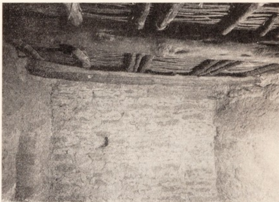
Ceiling, Spruce Tree Ruin.
