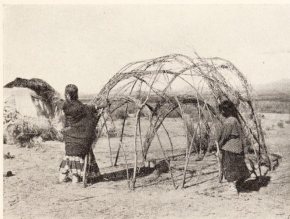
San Carlos Apache Women building a House.
