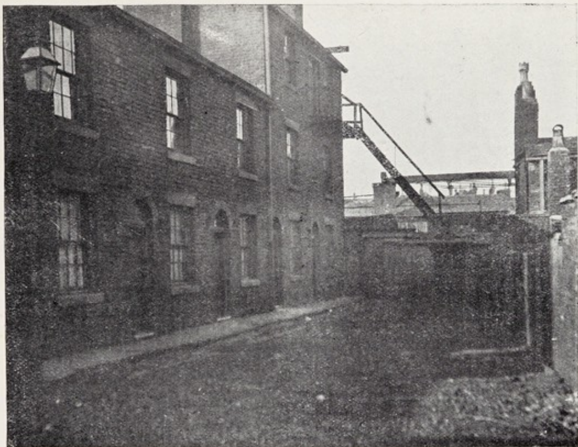
GILDING COURT (BEFORE ALTERATIONS), LOOKING SOUTH.
