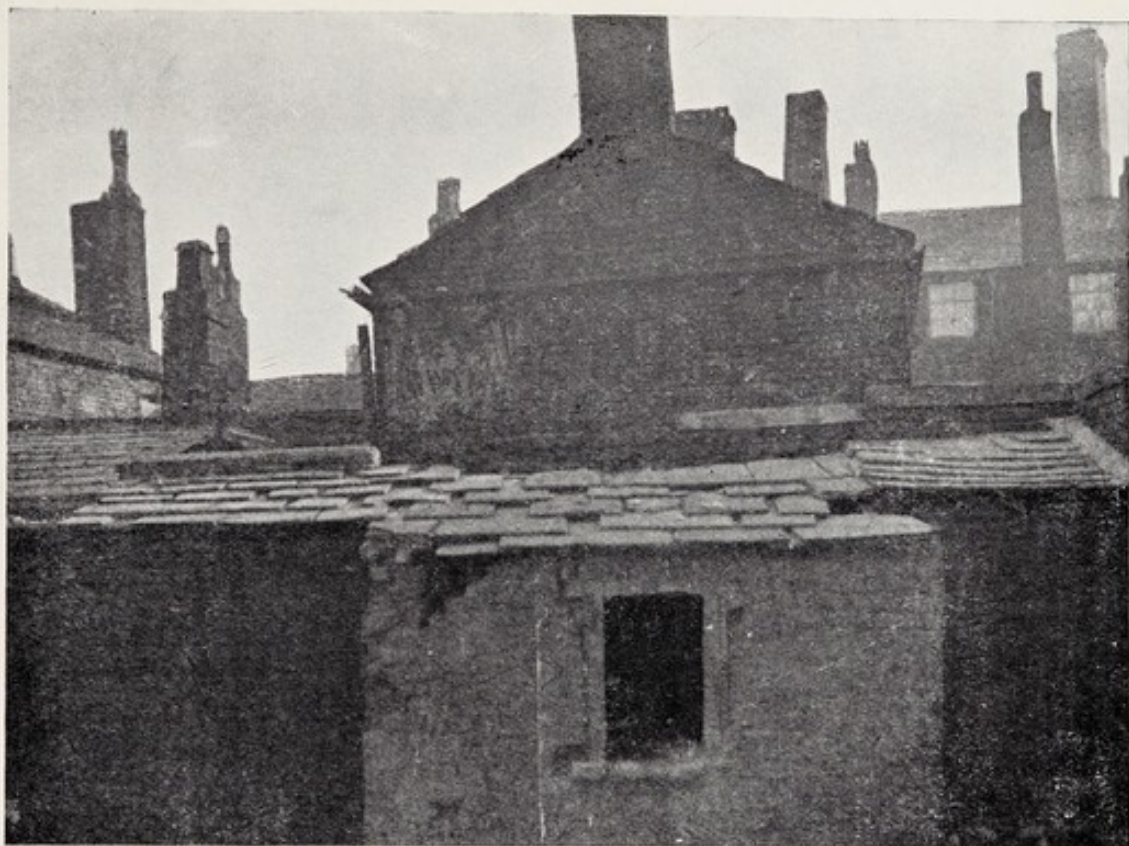
GILDING COURT (BEFORE ALTERATIONS), LOOKING NORTH.
