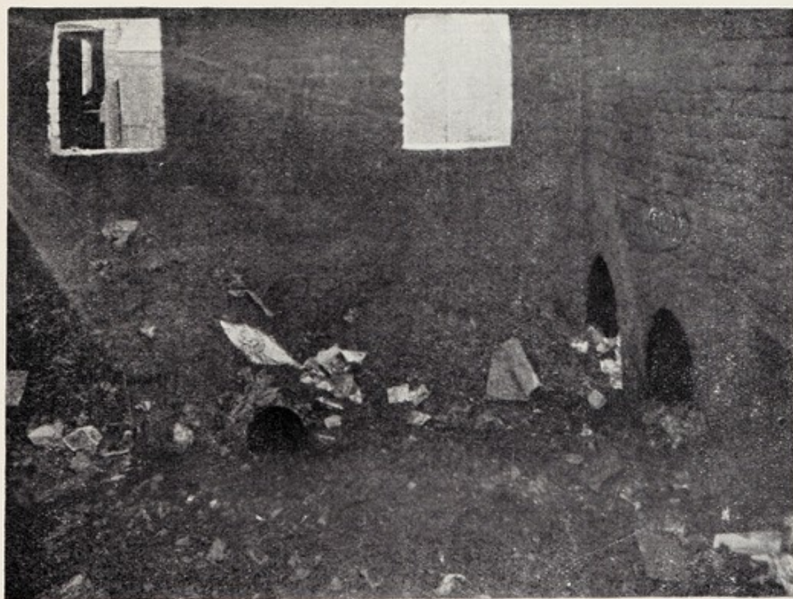
INTERIOR OF ASHPIT—" PIMHOLE CESS " (BEFORE ALTERATIONS).
