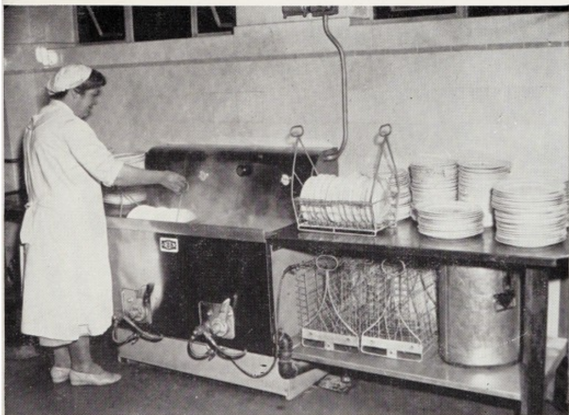
Plate II—Sterilising double sink used for washing of cutlery, crockery and dishes at an industrial canteen.
