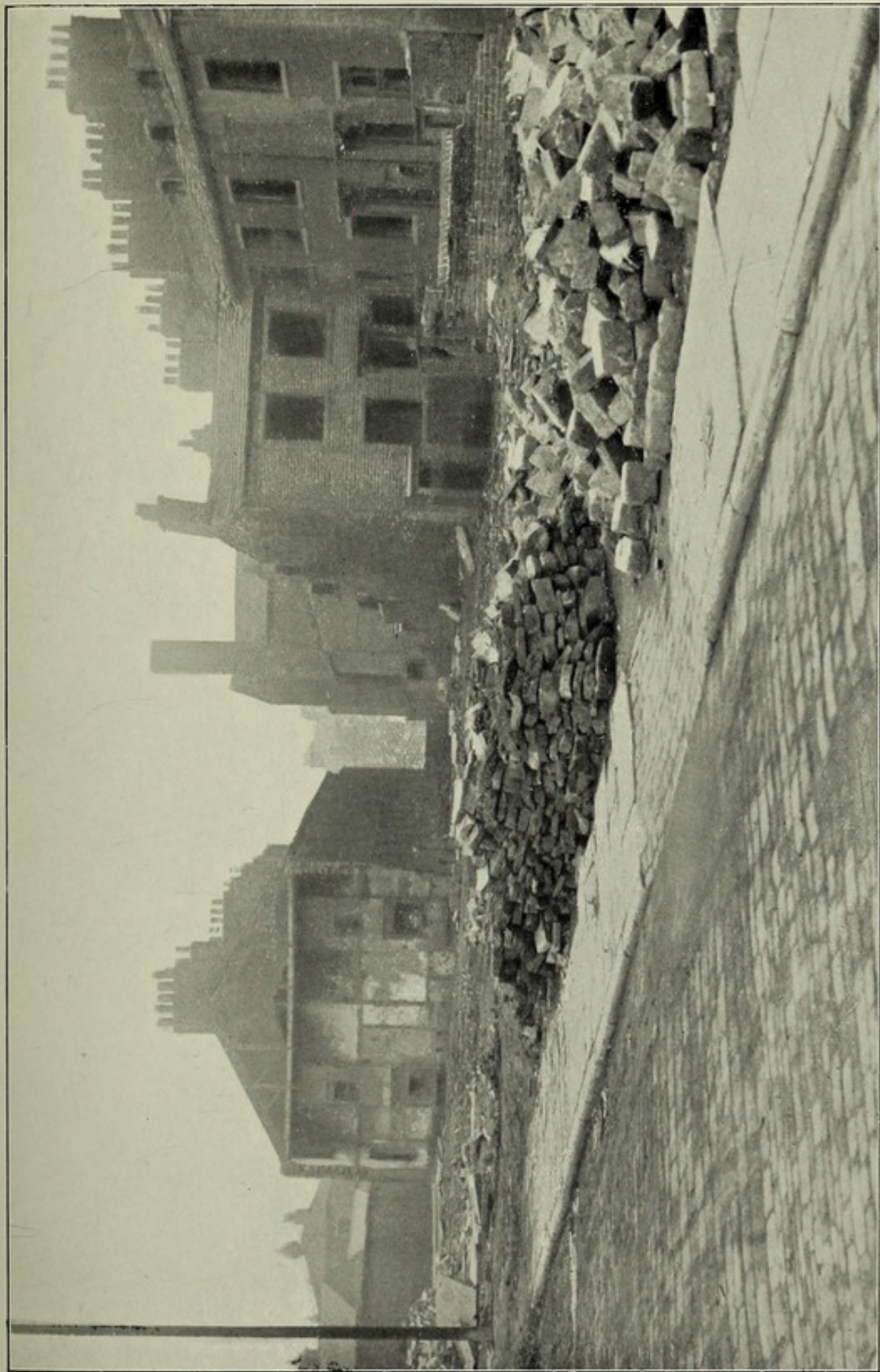
PHOTOGRAPH SHOWING THE DEMOLITION OF HOUSES ON THE SITE
