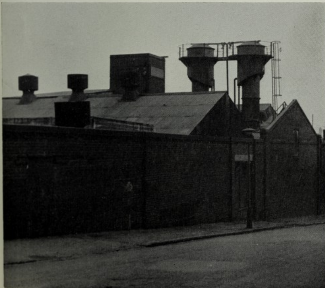
NO. 1a.—CUPOLAS : IMPROVED TYPE SHOWING WASHING ARRANGEMENTS
