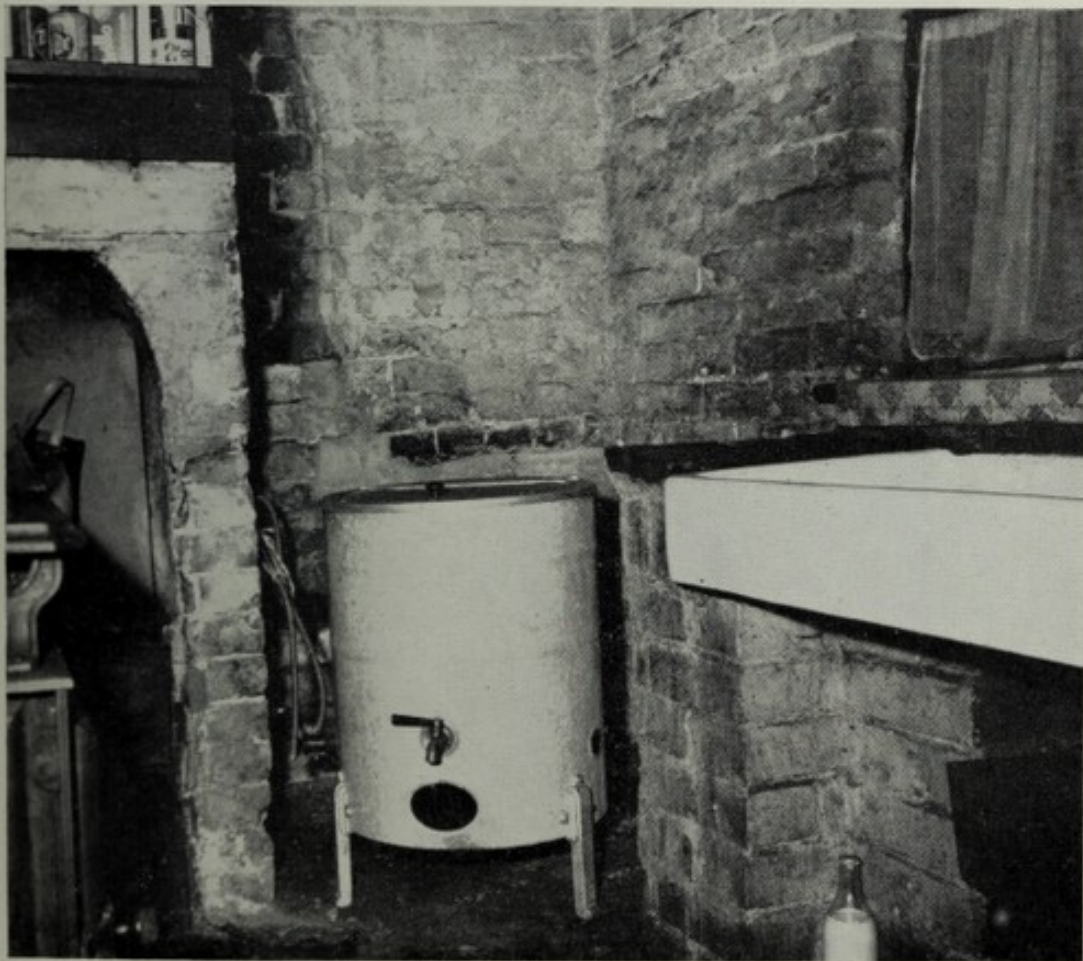
NO. 9—REPLACEMENT OF OLD TYPE SET-POT BY GAS WASH BOILER
