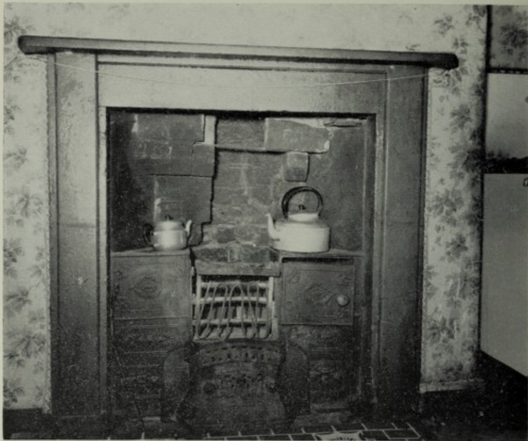
NO. 2.—OLD TYPE COAL BURNING RANGE BEFORE CONVERSION
