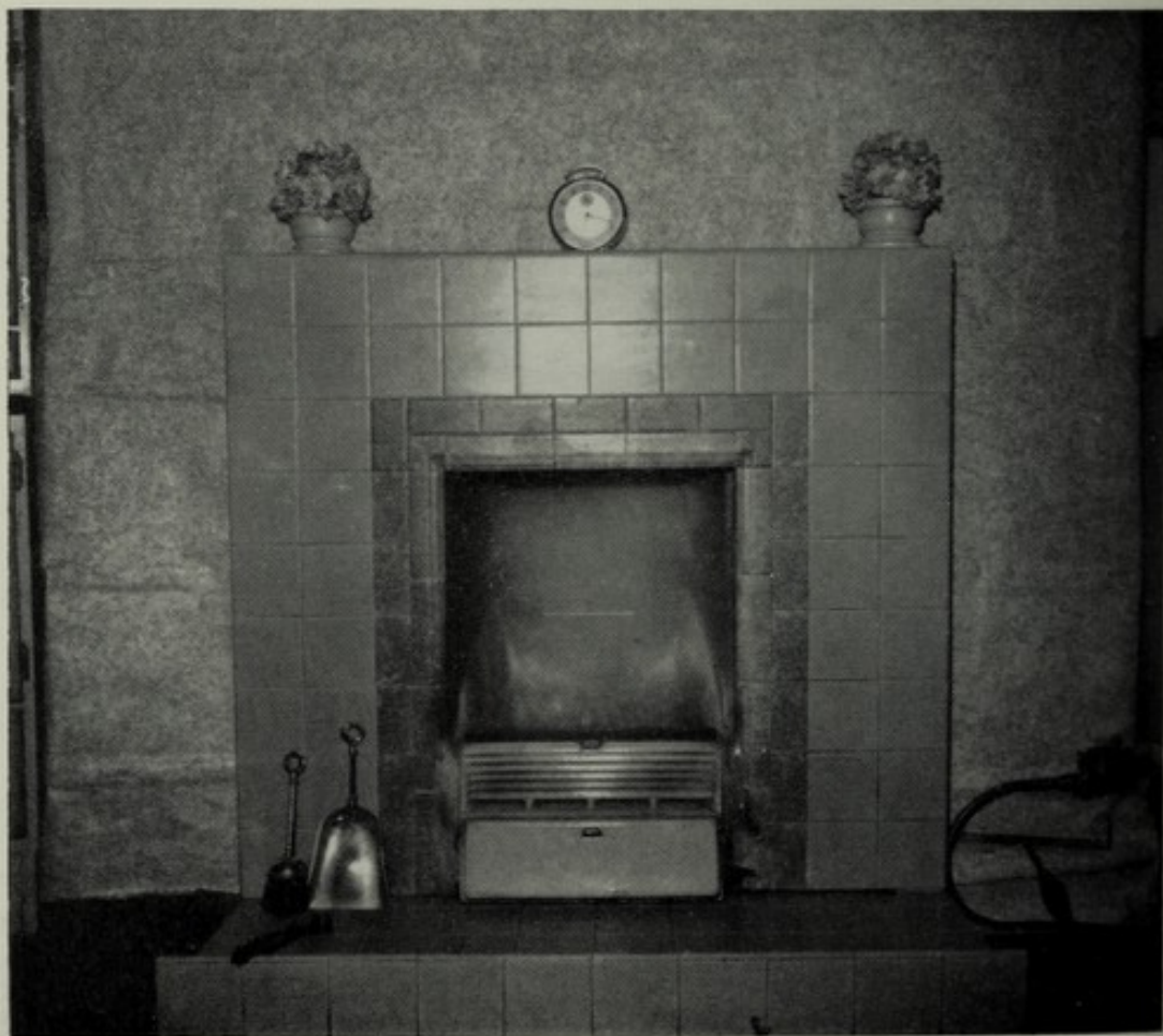
NO. 3.—CONVERSION OF OLD TYPE COAL BURNING RANGE BY A CONTINUOUS SOLID SMOKELESS FUEL BURNING FIRE WITH TILED SURROUND AND GAS IGNITION
