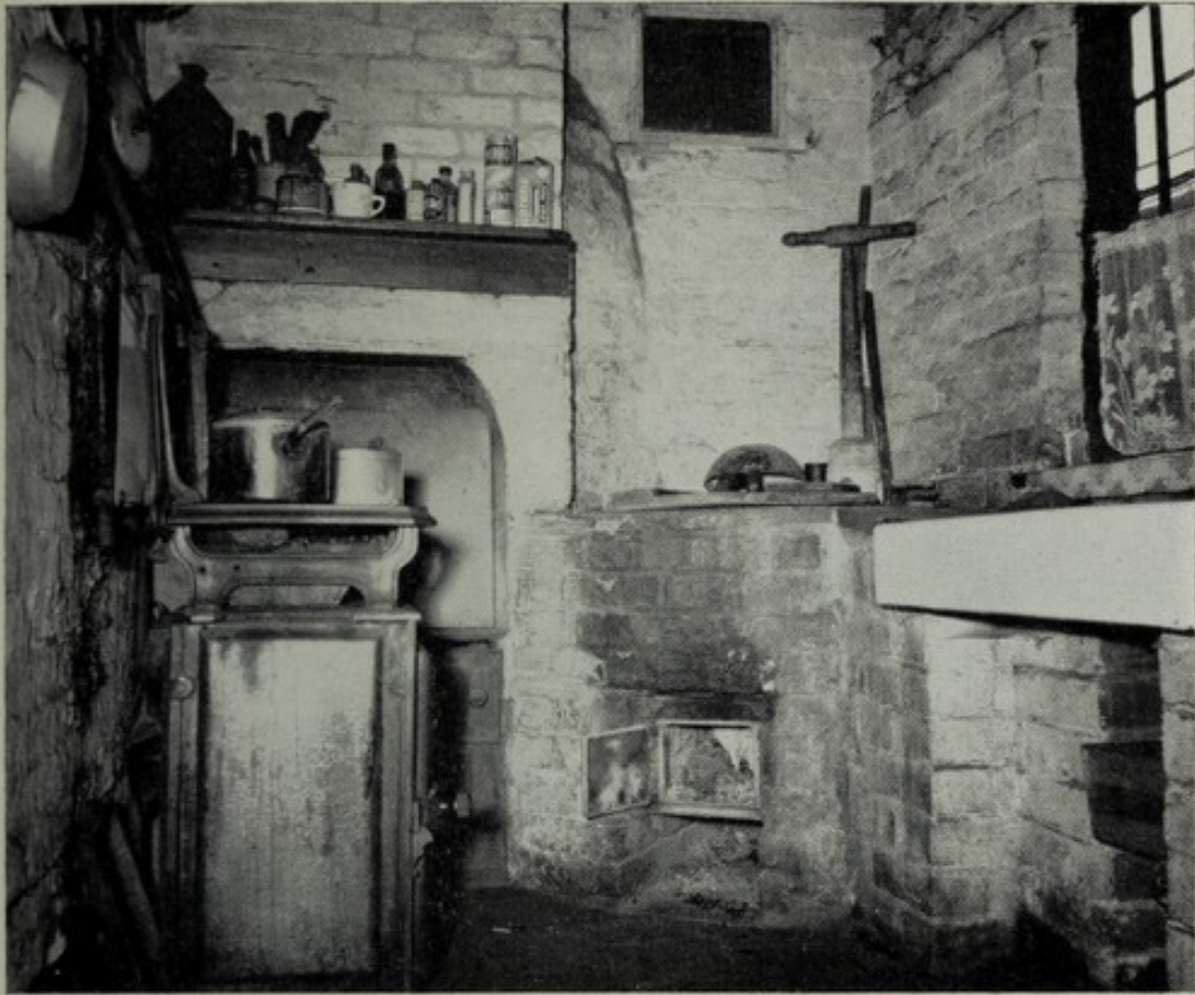
NO. 8—OLD TYPE SET-POT WASH BOILER BEFORE CONVERSION
