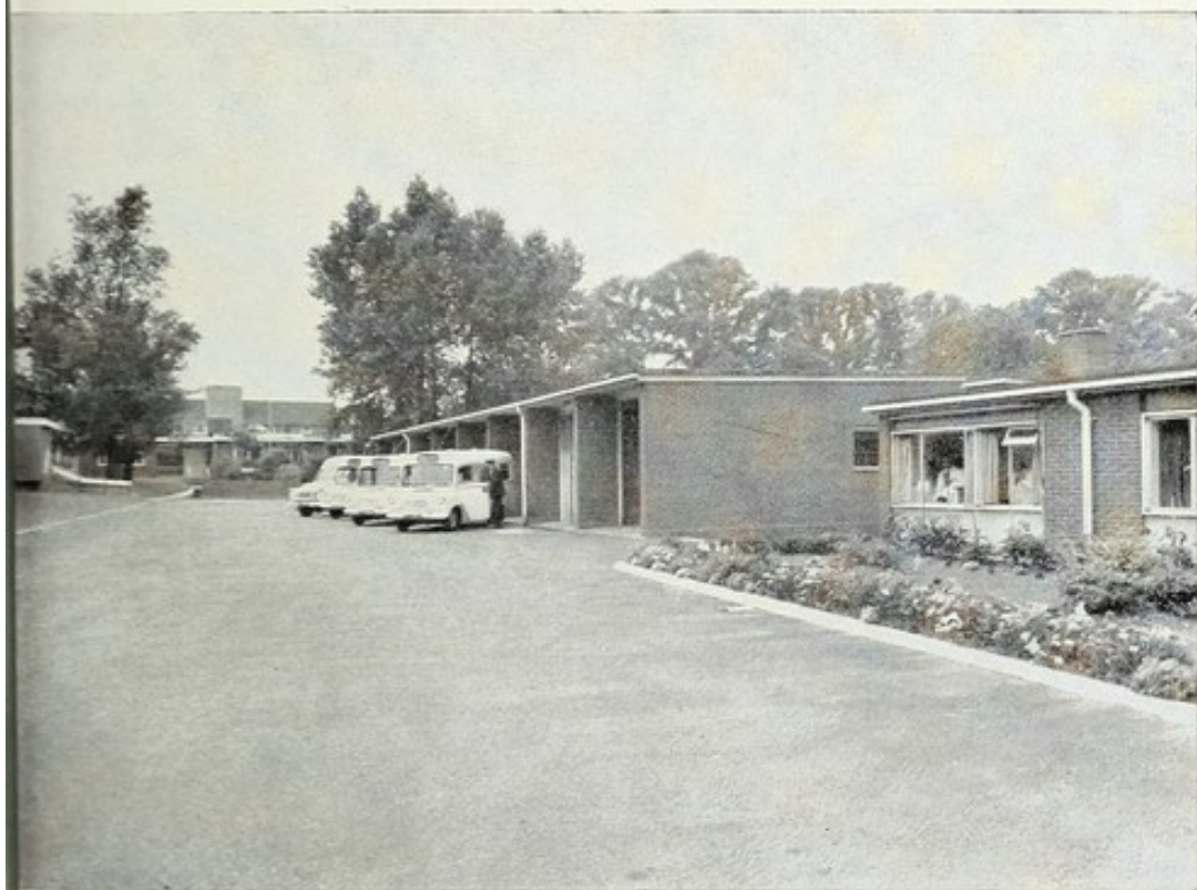
THE PATTERN OF THE NEW STATIONS WAS SET BY THE KEMPSTON AMBULANCE STATION.
