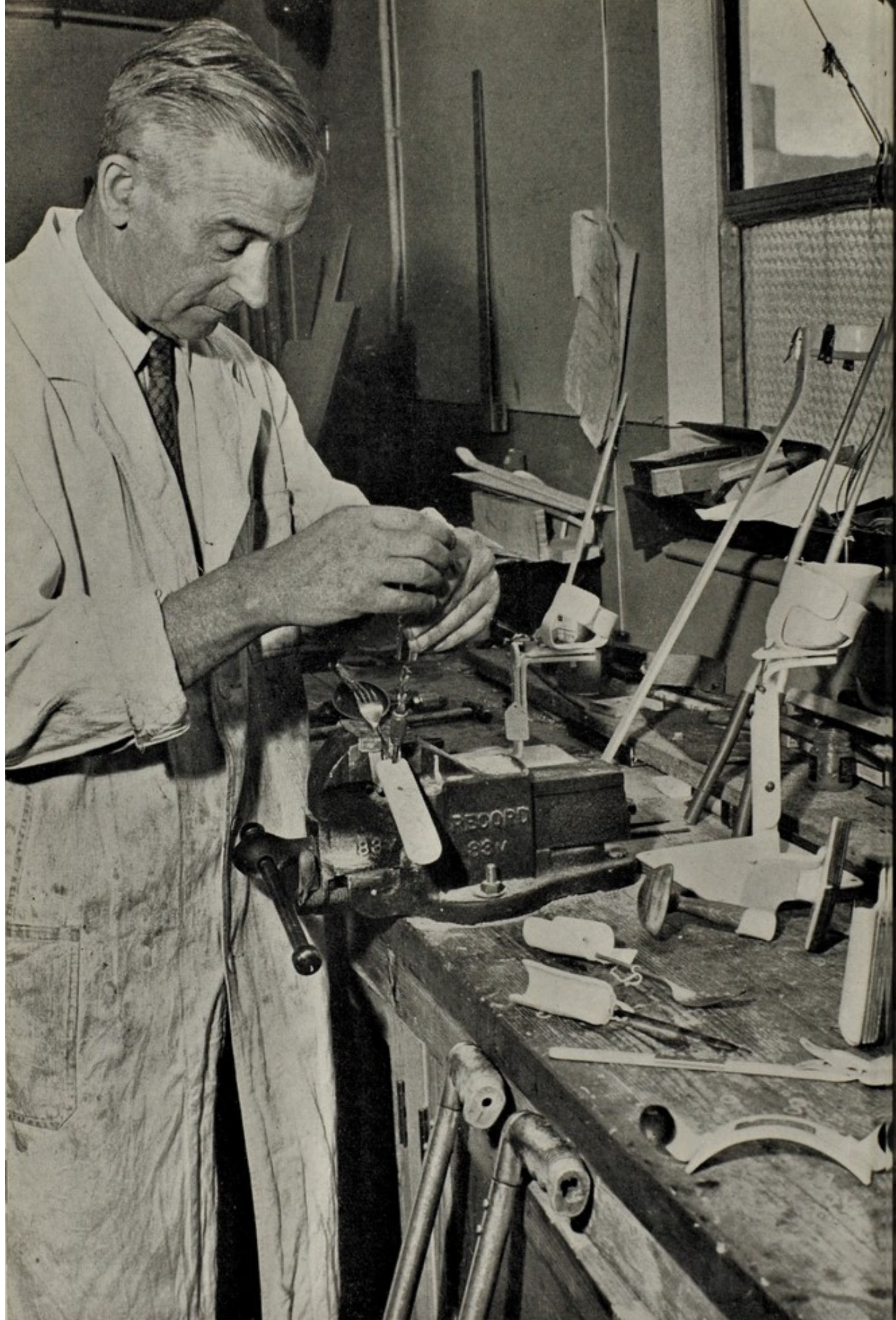
AIDS DEPARTMENT, COUNTY WORKSHOPS. CONSTRUCTION IN PROGRESS
