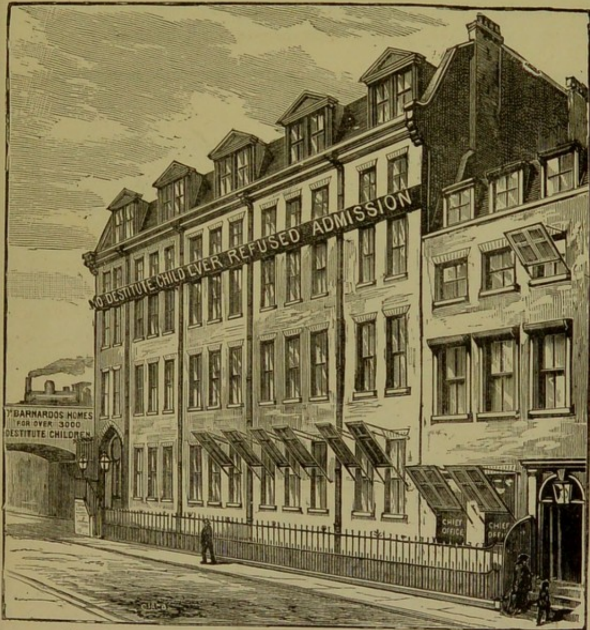
Front View of Central Offices and Boys' Home in Stepney Causeway.
