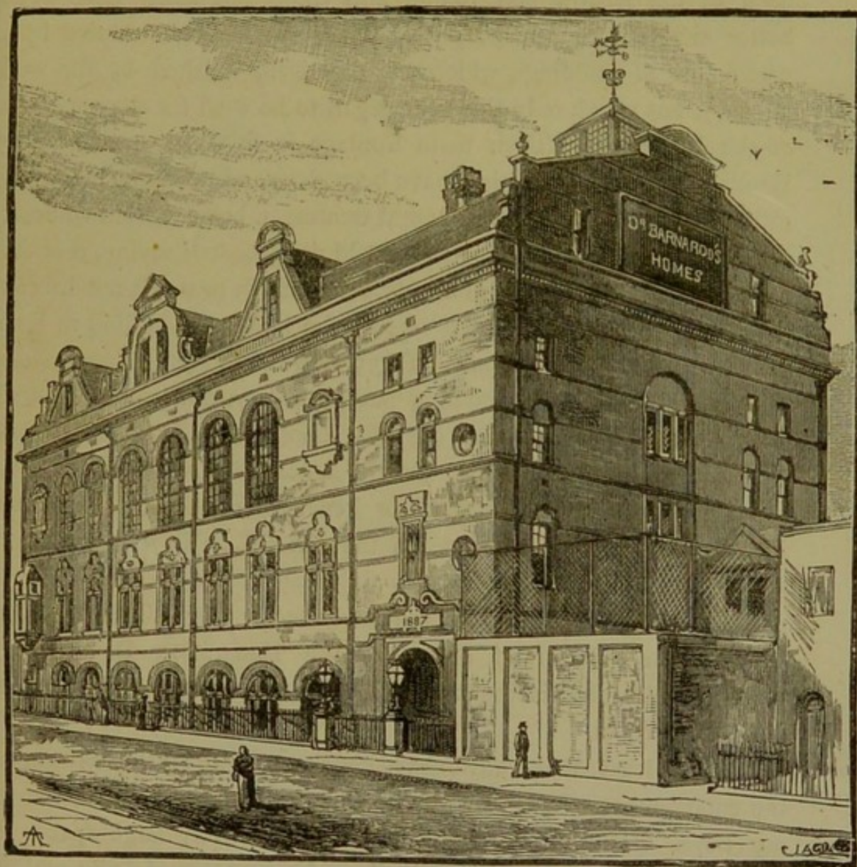
West Elevation of the Bower Street Addition, facing Bower Street.
