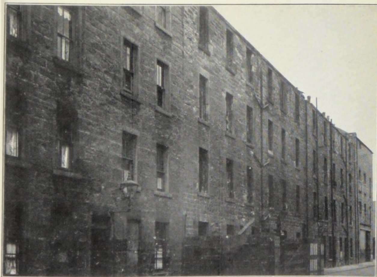
CLEARANCE AREA—EAST CROMWELL STREET.
