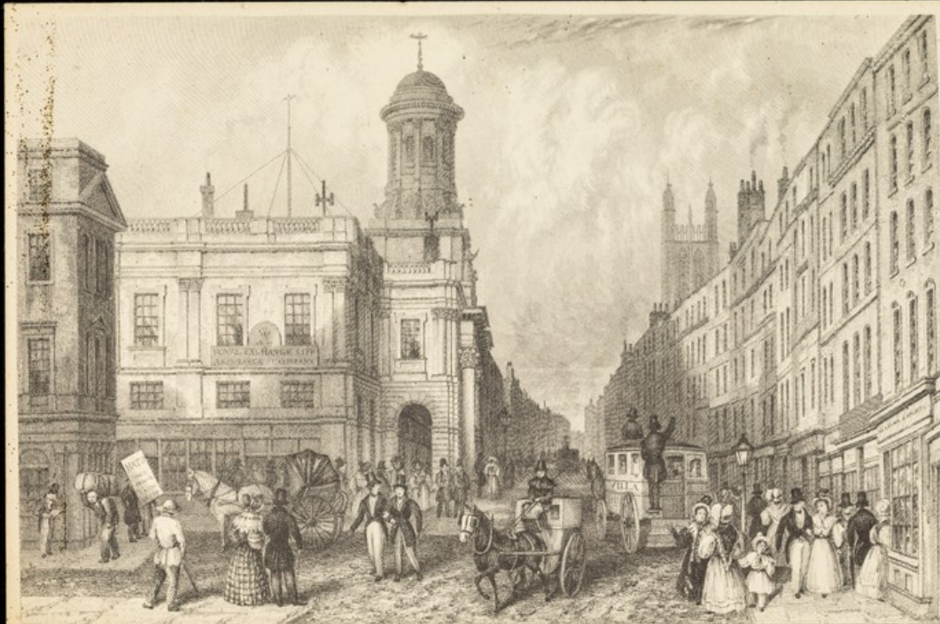
THE LATE ROYAL EXCHANGE AND CORNHILL. The tower of the Royal Exchange built by Jerman after the Great Fire of 1666, showed signs of weakness in 1821, and was taken down, to be replaced by the "pepper pot" shown in the picture. The whole building was destroyed by fire in 1838, in which year the view was probably taken. The Royal Exchange Assurance Company had its offices in the Exchange building, as it does today. Cornhill extends eastwards on the right, and activity in the street includes a street porter, a signboard man and an omnibus. The tower of the church of St. Michael, Cornhill, can be seen above the houses.
