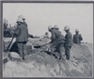
Sappers Covering Walls with Earth and Sand
