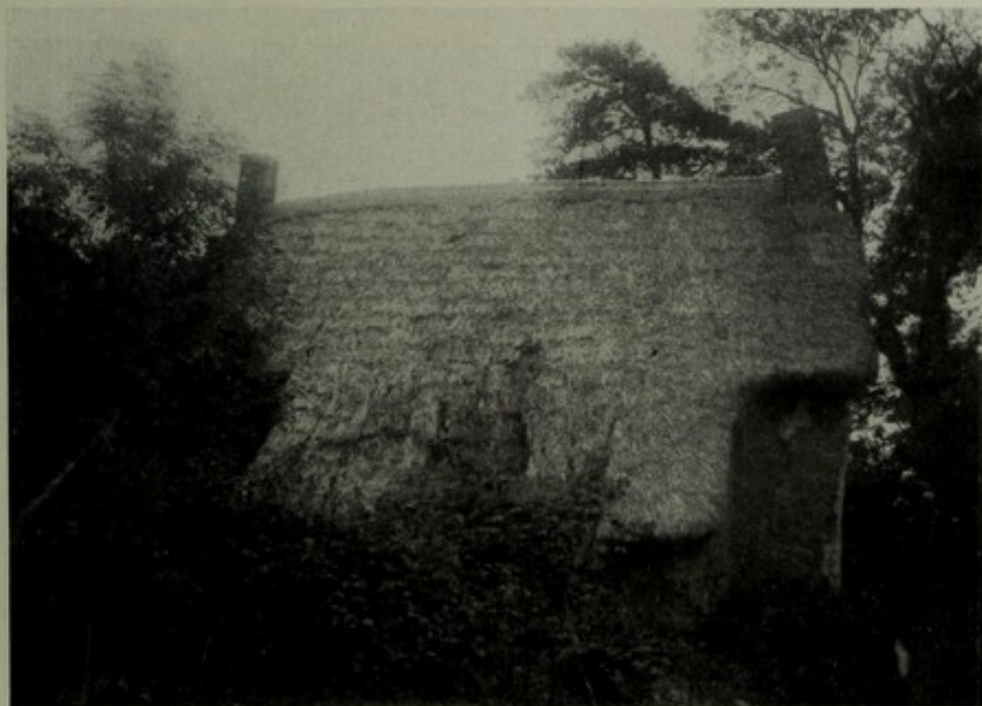
No. 2. Shows the back elevation of the "Hospital."
