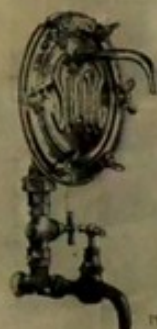
BP406 "Seitz-E.K." Water Sterilising Filter size 14/1.
