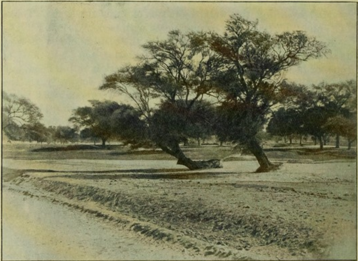
FIG. 1.—Tank "P." after completion of work. The water went beyond the trees. All the light portions of picture were formerly under water.
