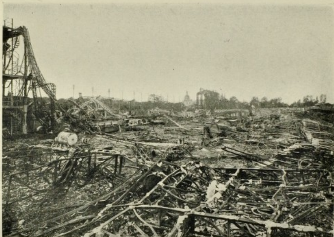
RUINS OF THE MAIN BUILDING SEEN FROM THE SE.
