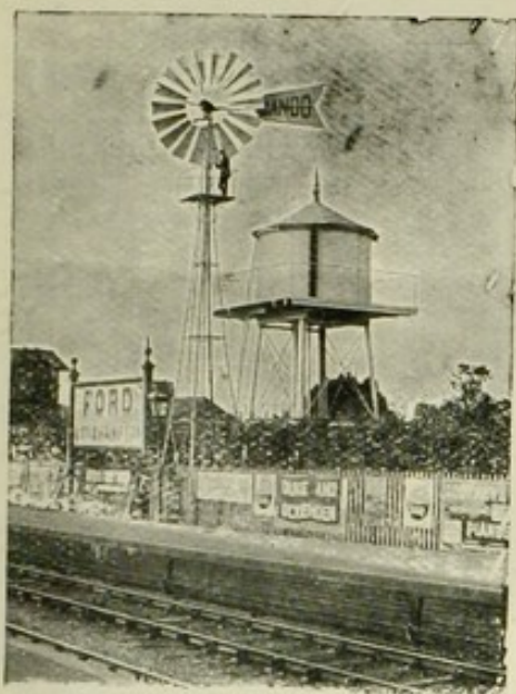
'Dando' Self-regulating Windmill with Reservoir.
