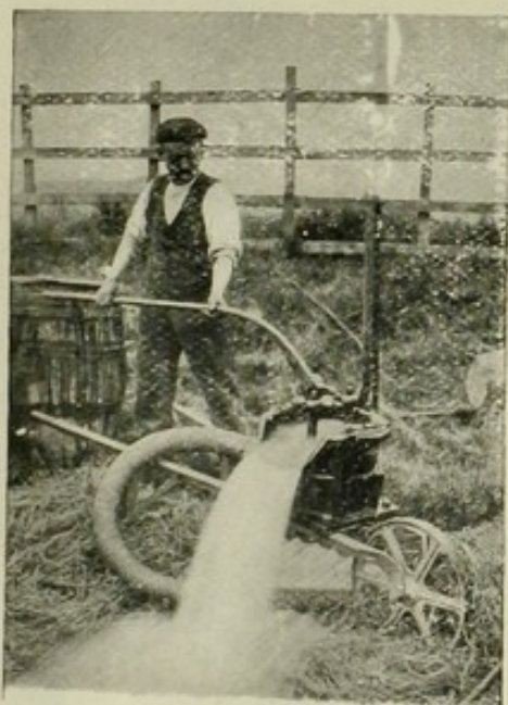
'Dando' Diaphragm Pump 3\frac{3}{4} 4000 gallons hour, for water and sewage.
