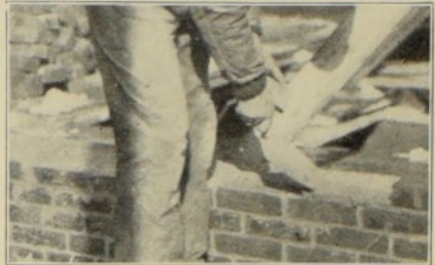
Fig. 29. — Spreading mortar on interior face tier.
