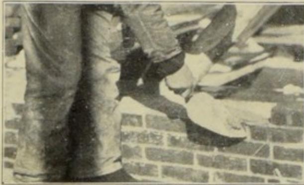
Fig. 30. — Cutting off mortar before brick is laid.
