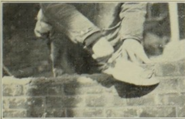
Fig. 36.—Working left to right.—Cutting off mortar after brick is laid on exterior face tier.
