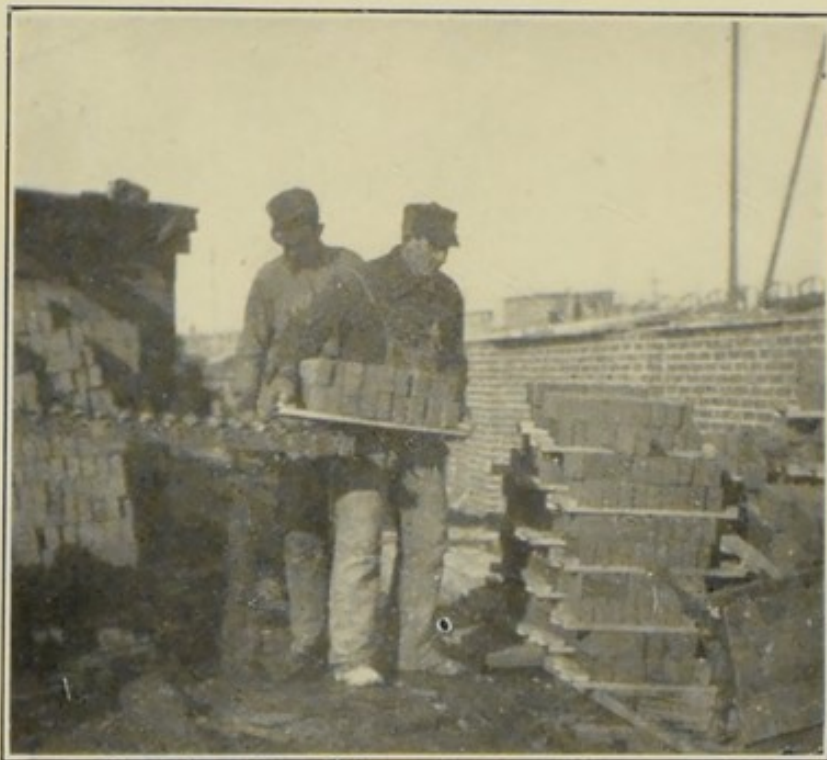
Fig. 3.—Arrangement of gravity conveyor for unloading brick so that laborer does not have to stoop.
