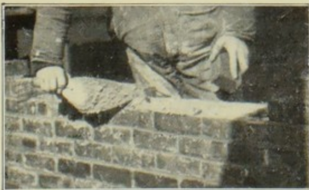
Fig. 26. — Buttering the end of the laid brick on the exterior face tier.
