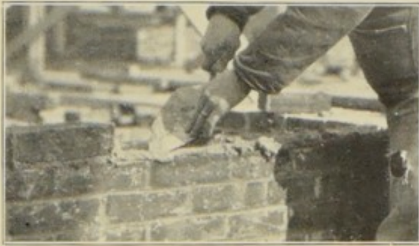
Fig. 40.—Working left to right.—Spreading mortar on the interior face tier.
