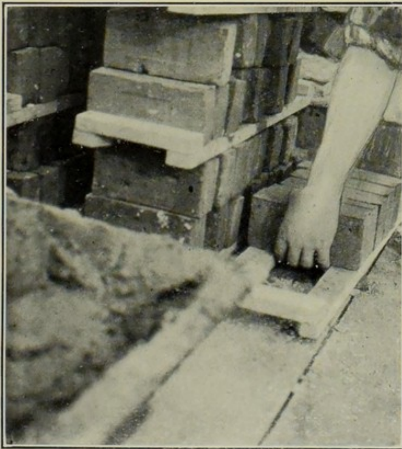
Fig. 6. — Right way to pick up brick from the lower tier on the packet.
