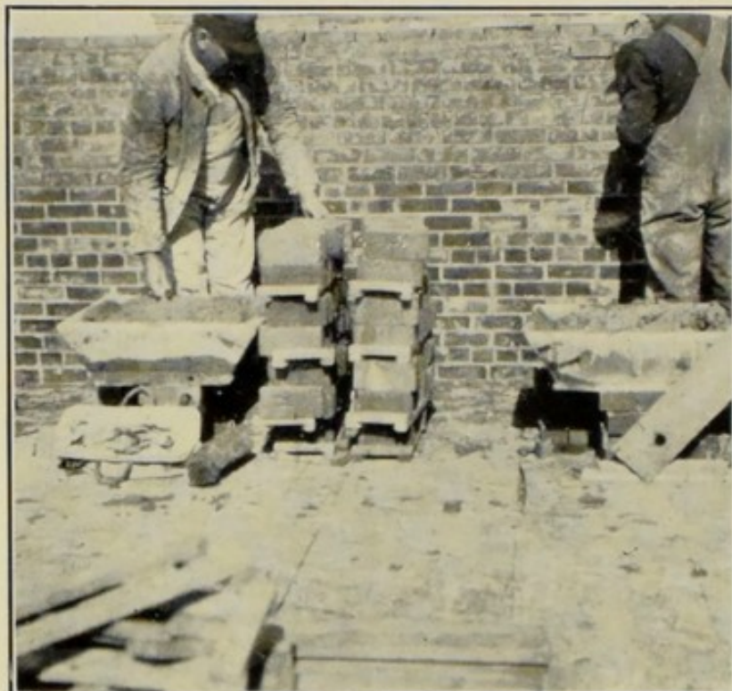
Fig. 12. — Standard practice for providing bricklayers with material for pick-and-dip method of bricklaying when the wall is shoulder high.
