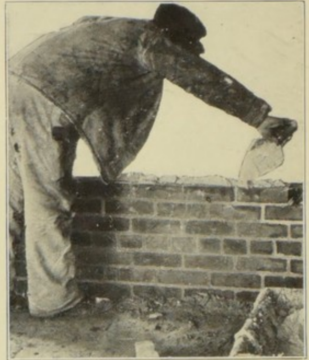
Fig. 41.—Working left to right.—Throwing mortar on the interior face tier.
