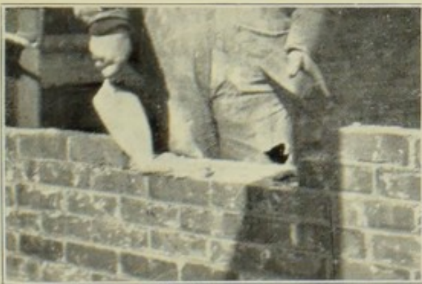
Fig. 24. — Spreading mortar on exterior face tier.
