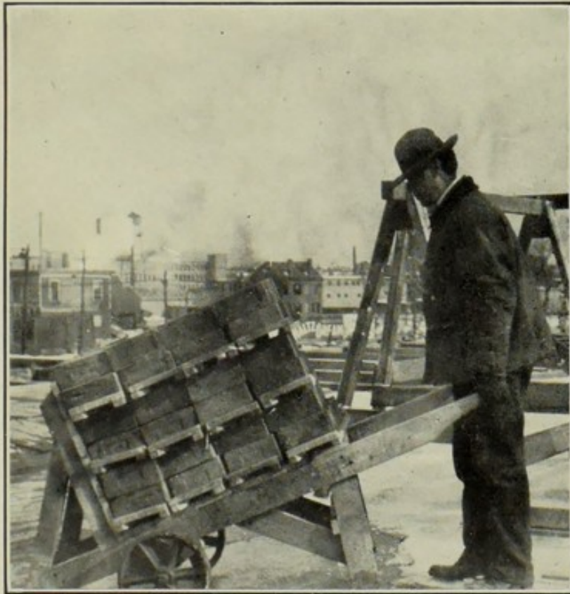
Fig. 20. — The two-wheeled trucket for carrying 12 packs. This trucket is so perfectly balanced that it causes less fatigue than the ordinary wheel-barrow.
