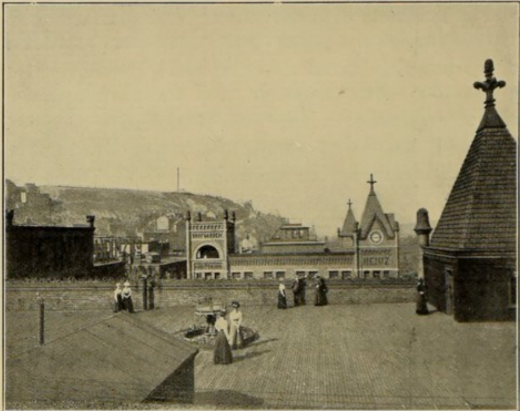
PART OF ROOF GARDEN ON MESSRS. HEINZ' FACTORY.
