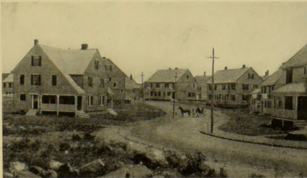
NEW PART OF HOPEDALE IN COURSE OF ERECTION.
