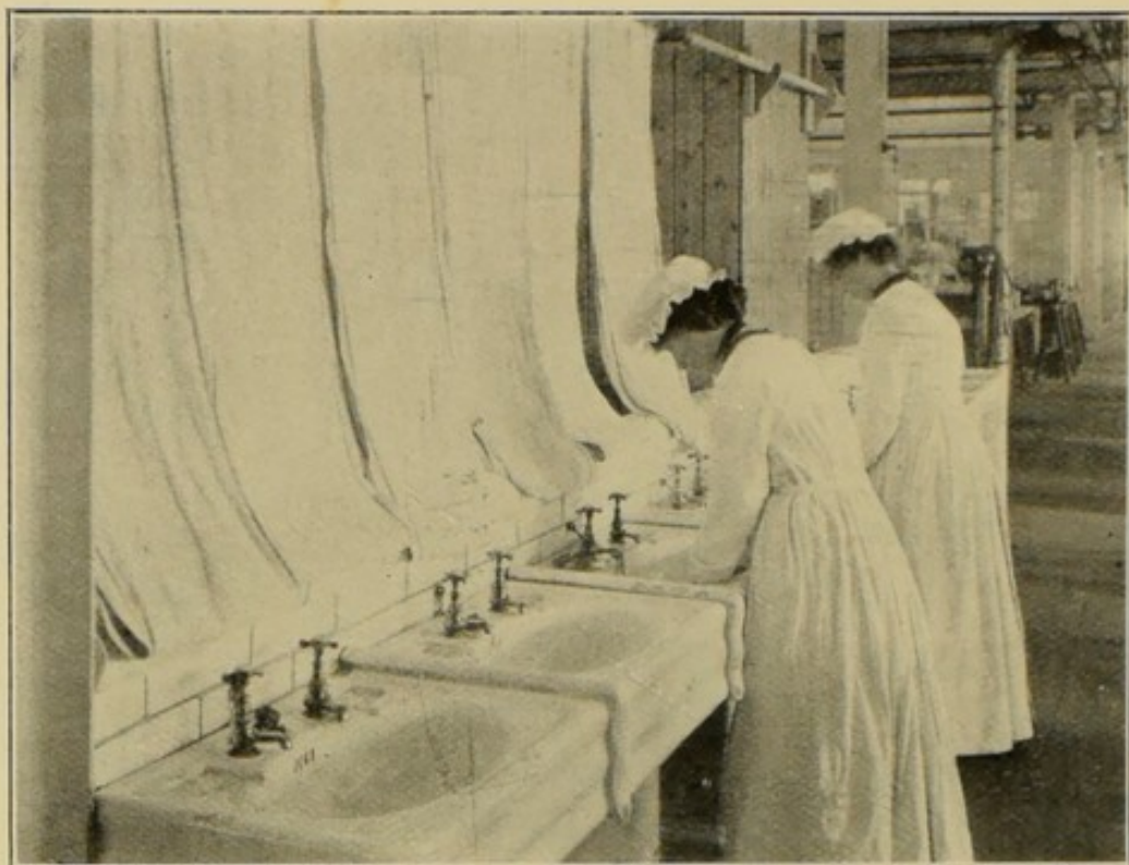
SANITARY ACCOMMODATION AT THE TABLOID WORKS.
