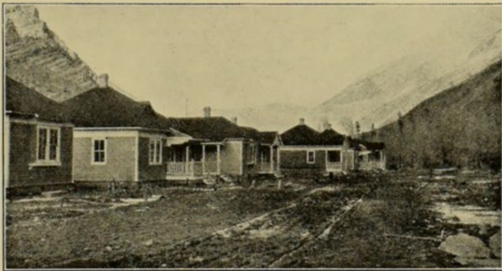
HOMES BUILT BY COLORADO FUEL AND IRON COMPANY IN PLACE OF SHANTIES.
