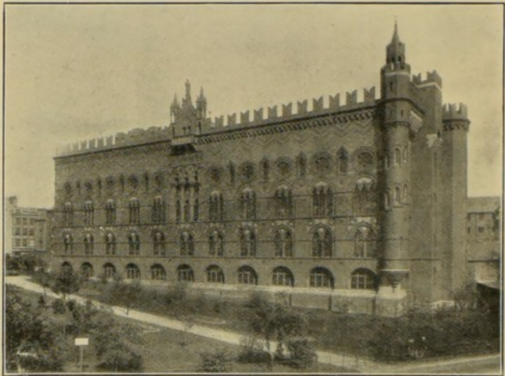
FAÇADE OF MESSRS. TEMPLETON'S FACTORY.
