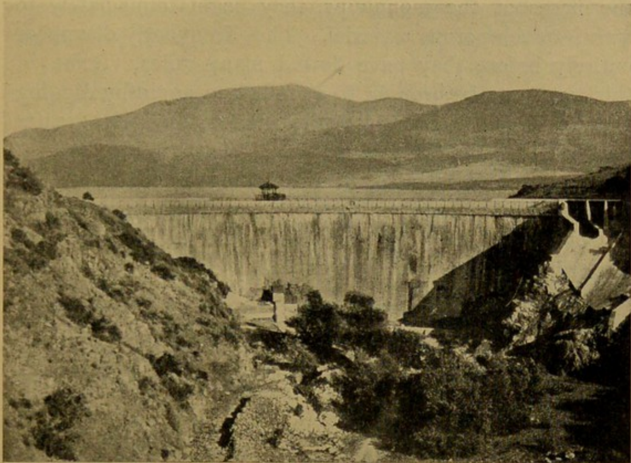
FIG. 116. — SWEETWATER RESERVOIR, NEAR SAN DIEGO, CALIFORNIA
