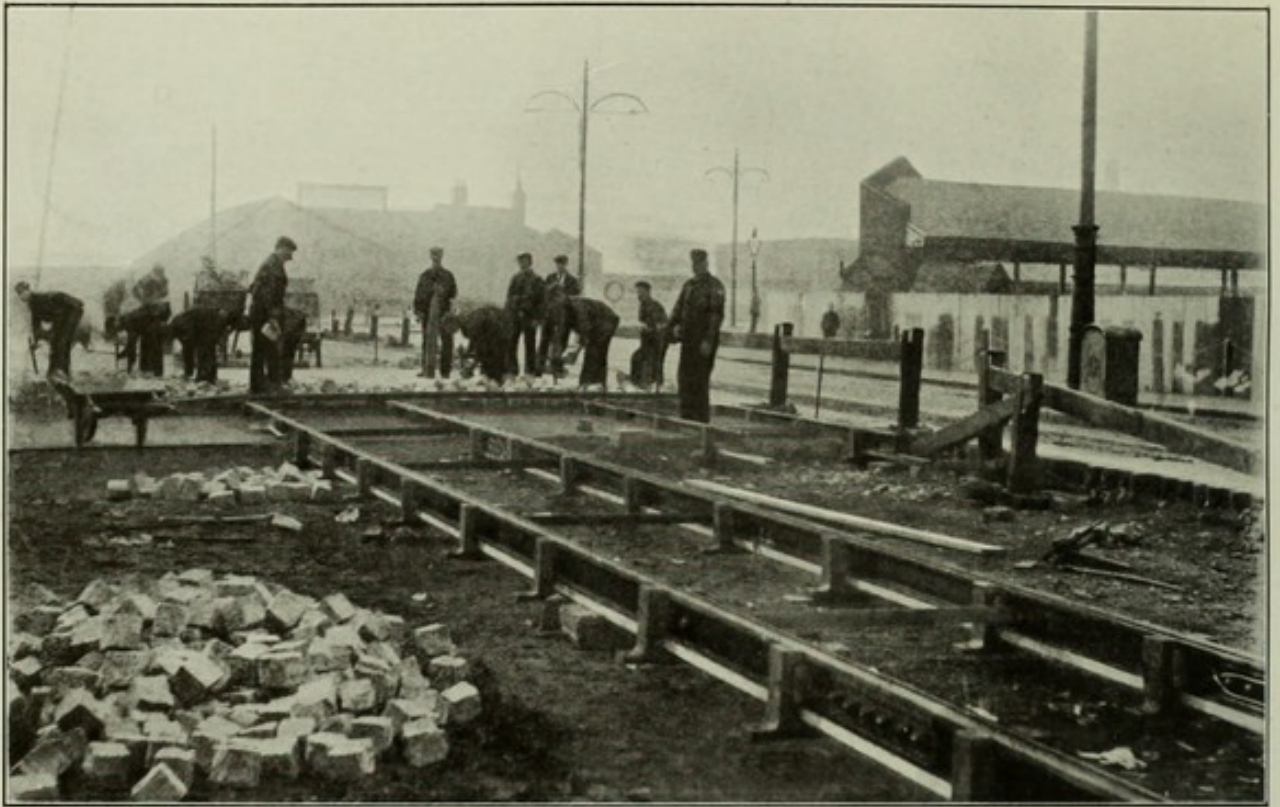
VIEW OF TRAMWAY IN COURSE OF CONSTRUCTION.
