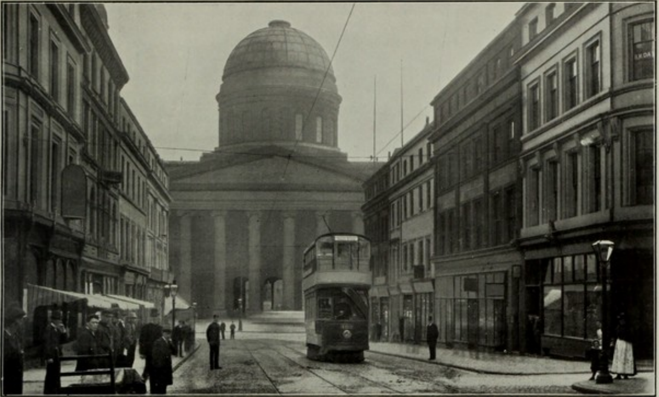
SPAN WIRE, WITH ROSETTE CONSTRUCTION, SOUTH CASTLE STREET.
