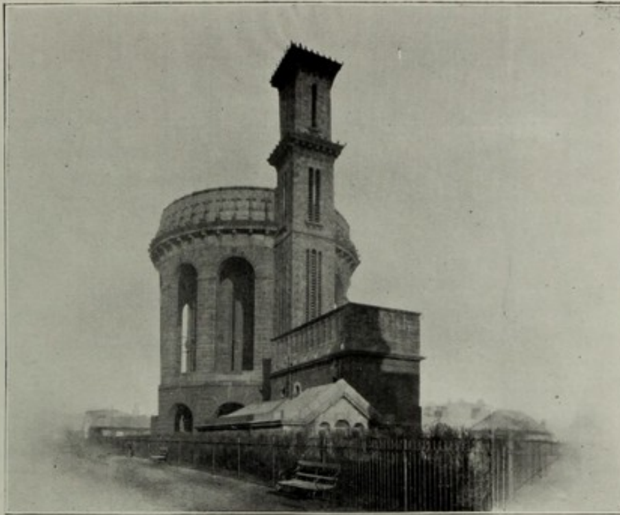
HIGH LEVEL PUMPING STATION, AUBREY STREET.
