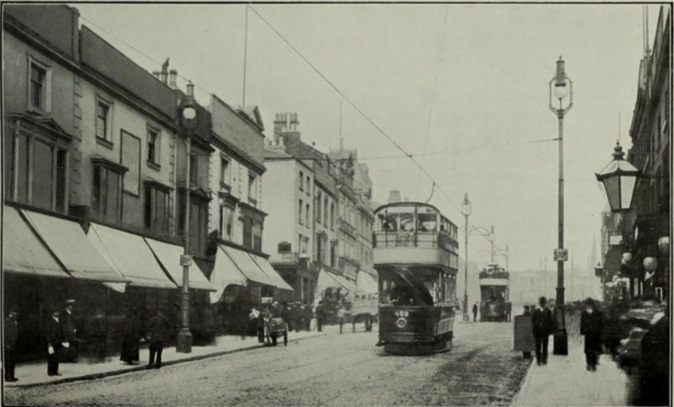
SPAN WIRE, WITH SIDE POLE CONSTRUCTION, LONDON ROAD.
