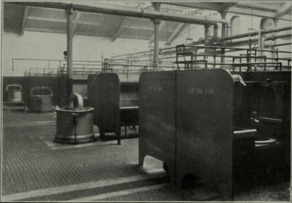
BURROUGHS GARDEN PUBLIC WASH-HOUSE.
