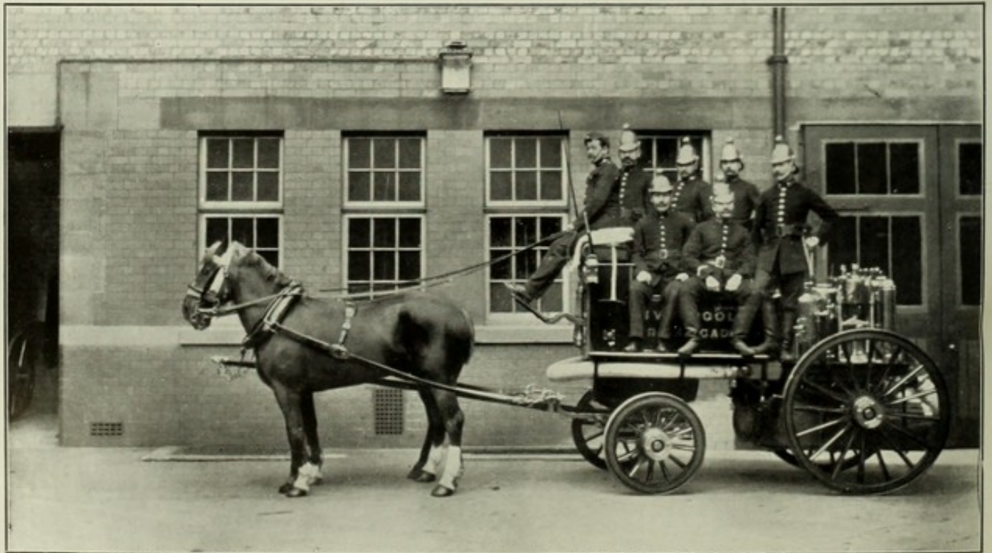
LIVERPOOL FIRE BRIGADE STEAM FIRE ENGINE "MAXWELL" PUMPS 450 GALLONS PER MINUTE
