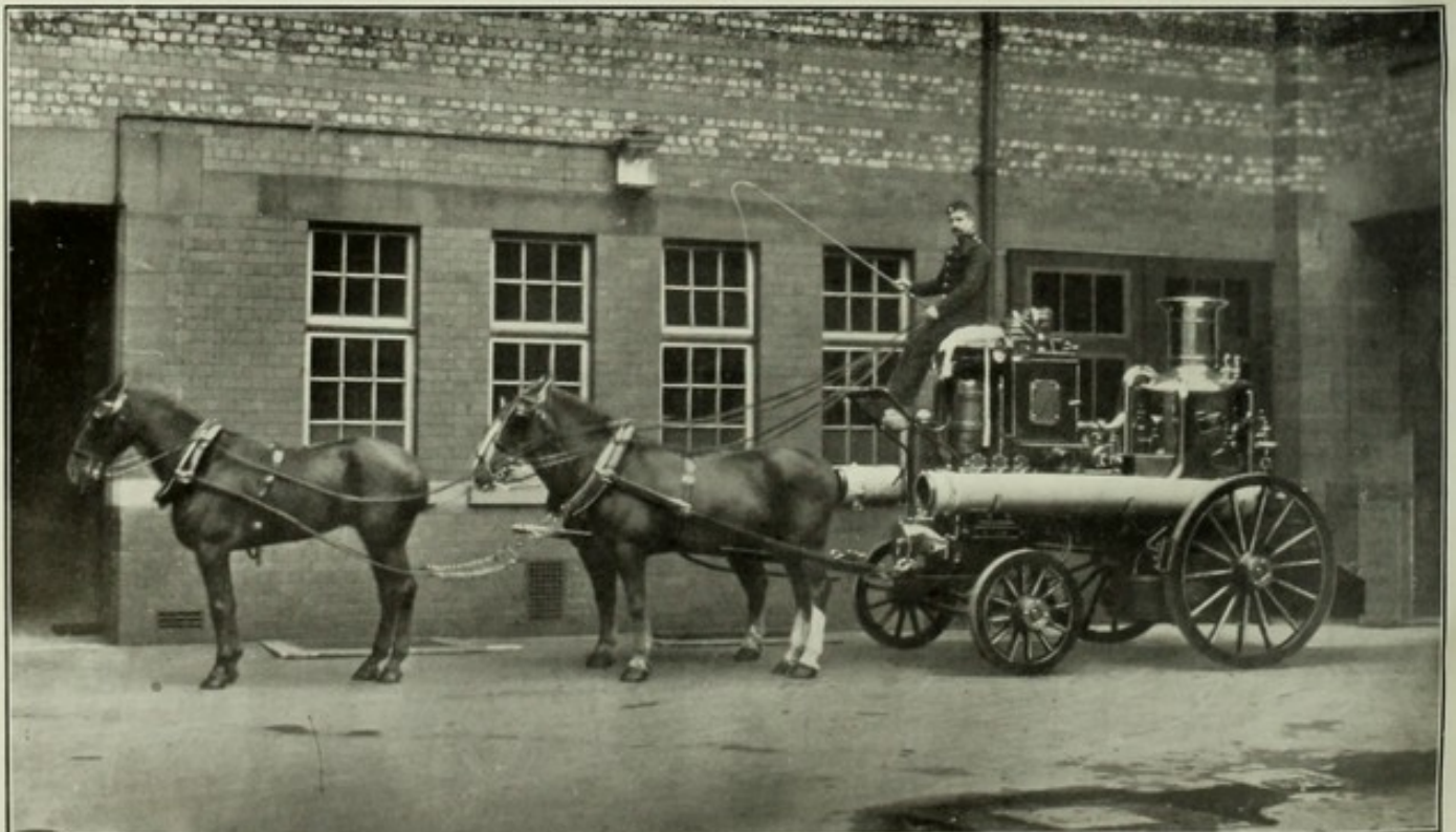
LIVERPOOL FIRE BRIGADE STEAM FIRE ENGINE "HOLT." PUMPS 1,800 GALLONS PER MINUTE.
