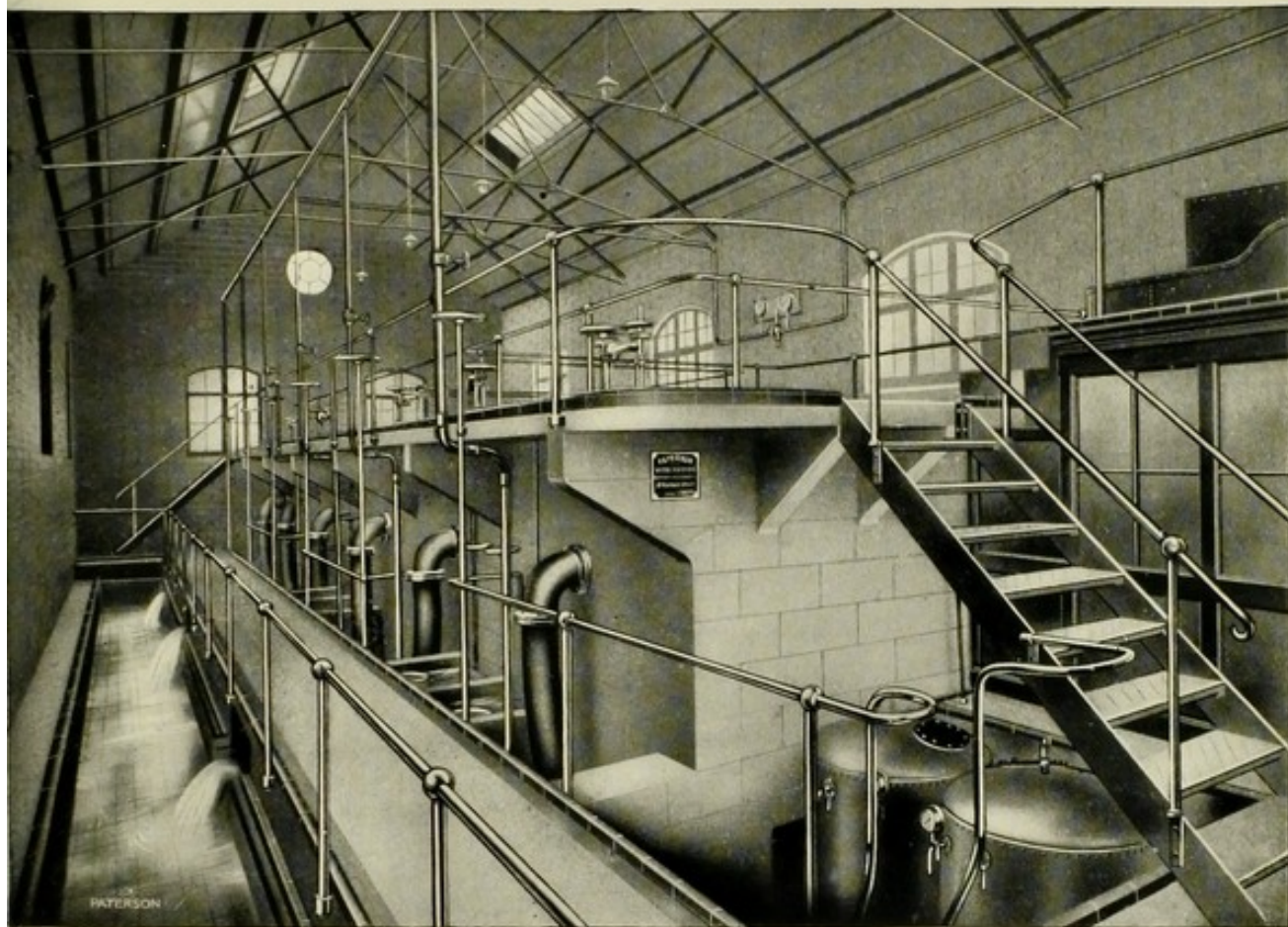
INSTALLATION OF RAPID FILTERS AT TEWKESBURY, PATERSON SYSTEM.
