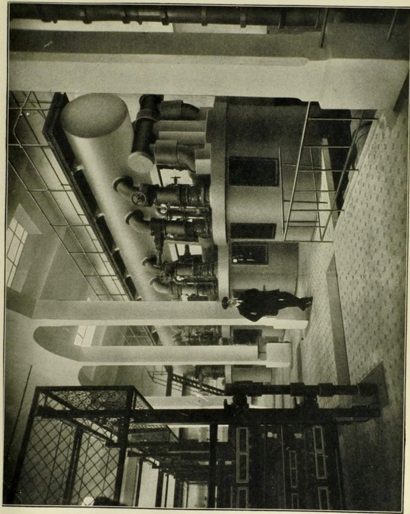
STERILISING TOWERS AND OZONE EMULSIFIERS, PETROGRAD.
