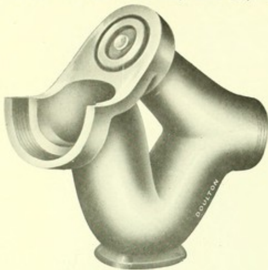
Fig. 66—SEWER-GAS INTERCEPTOR. With inspection arm and air-tight stopper.
