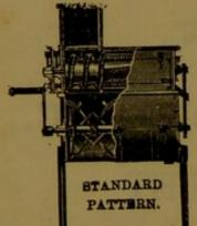
Is a Perfect Machine for Reducing, Sifting, and Mixing all kinds of Dry and Lumpy Powders at one operation, without creating dust.
