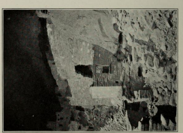
has a large front window and two smaller openings higher up in the second story of the western wall. The combined front walls of rooms 17 and 18 may be ranked among the finest examples of masonry in Cliff Palace. The large embrasures made in this wall by vandals were repaired.
