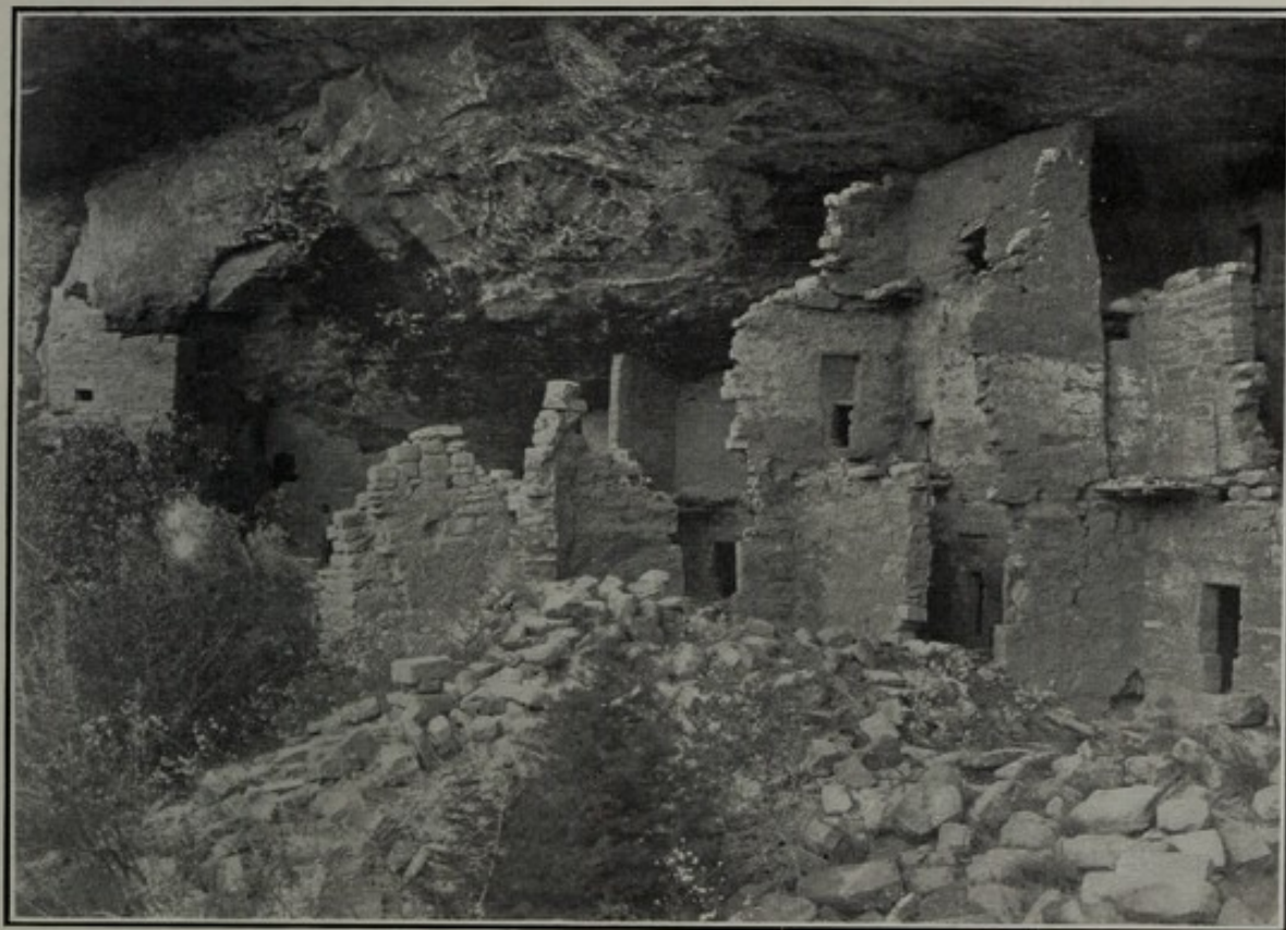
Plaza E, from the south, before repair
