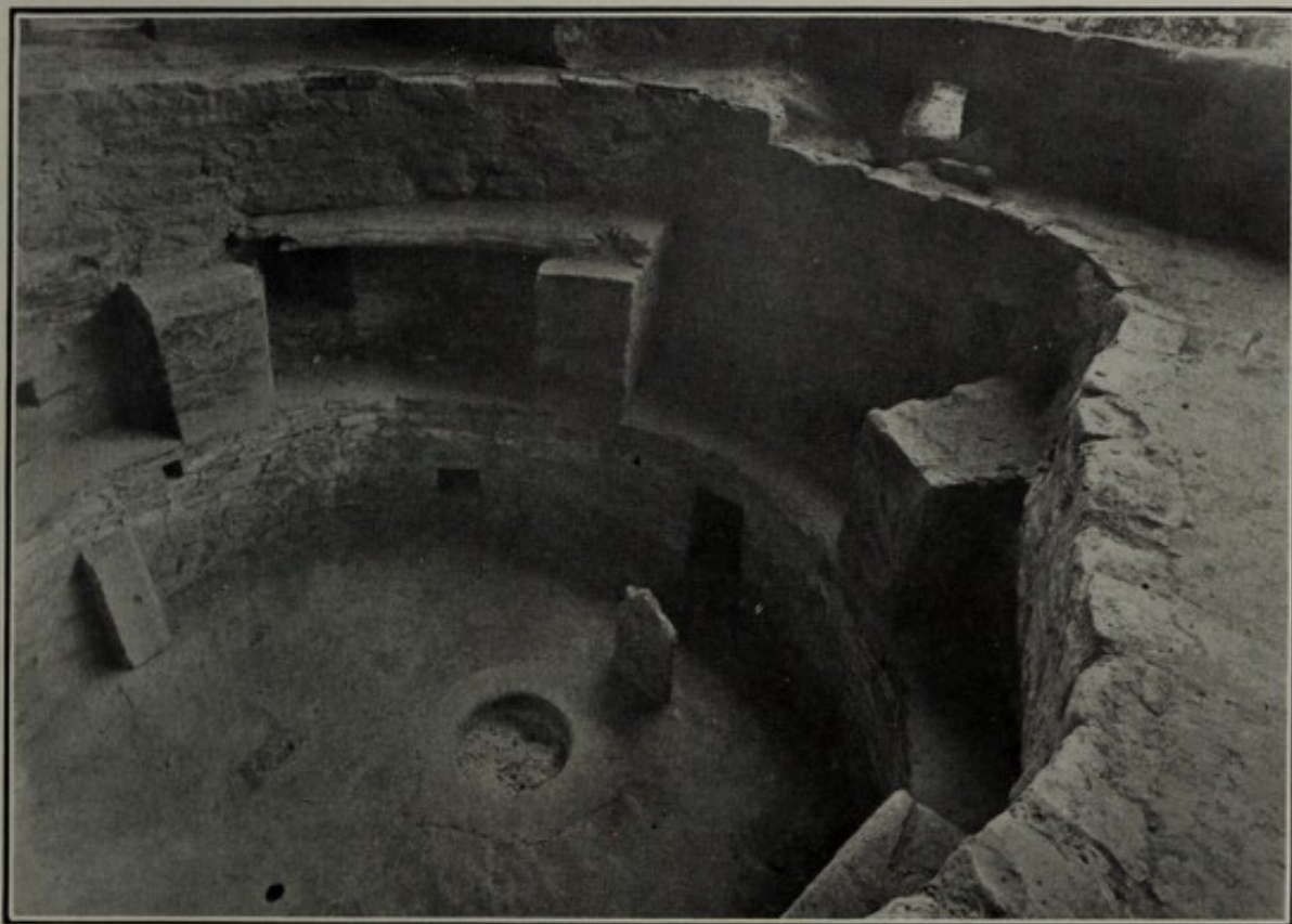
Kiva D, repaired
