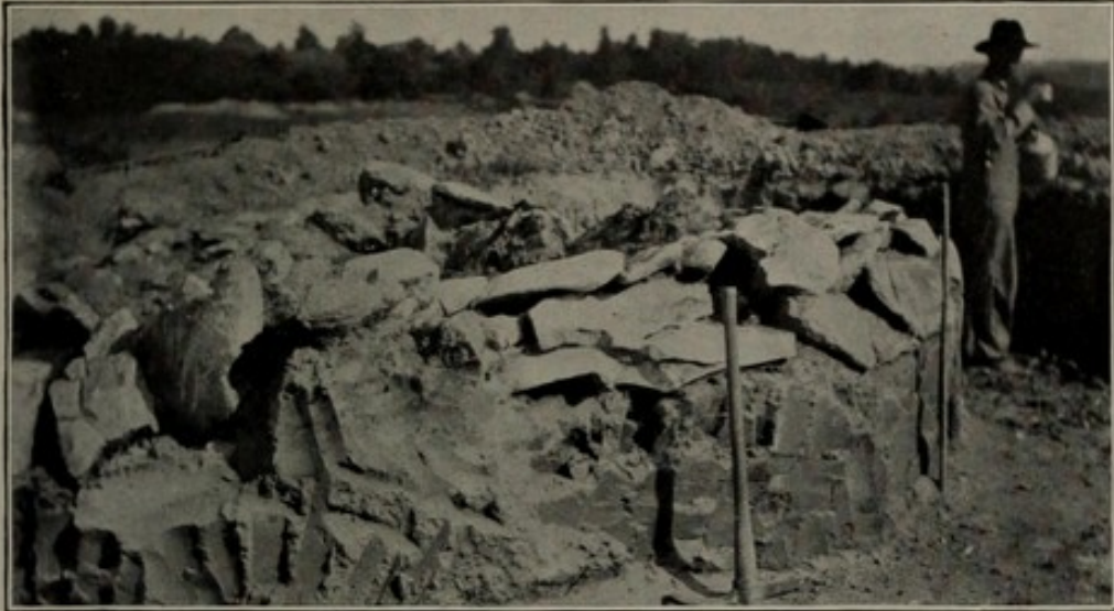
a EXTERIOR OF VAULT
