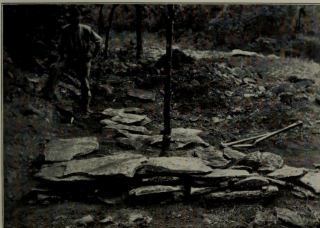
b LOOKING ALONG THE EAST SIDE OF THE LOUISIANA WORK
