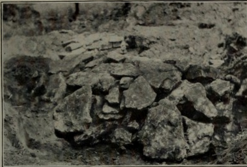
a OUTSIDE AND TOP OF WEST WALL IN MOUND NO. 2
