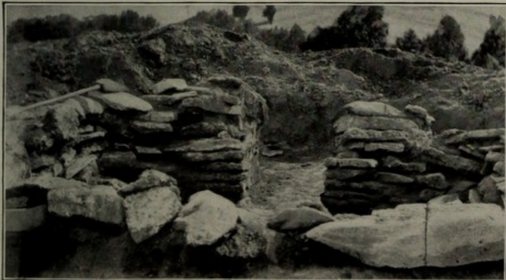
c DOORWAY IN VAULT
