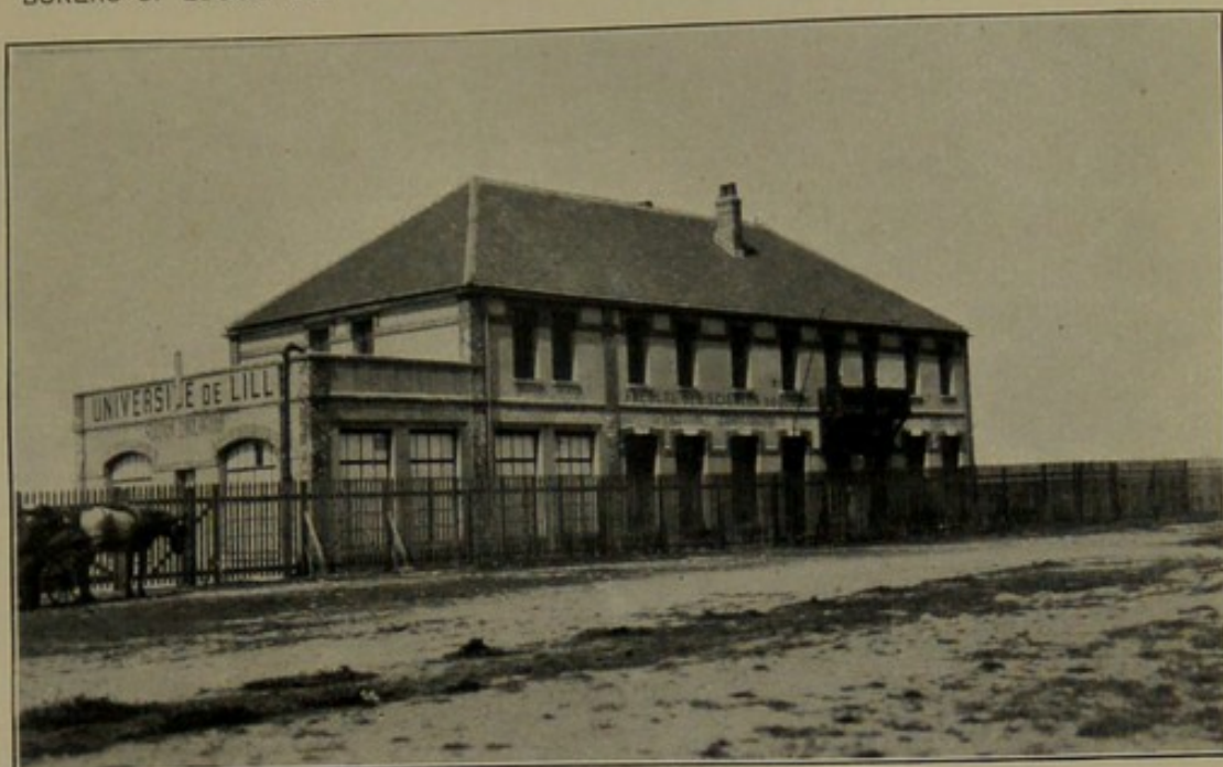
A. STATION BUILDING.
