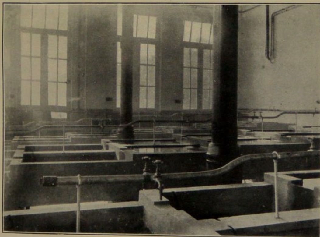
B. INTERIOR OF RESEARCH AQUARIUM ROOM, SHOWING BANKS OF CEMENT TANKS.
