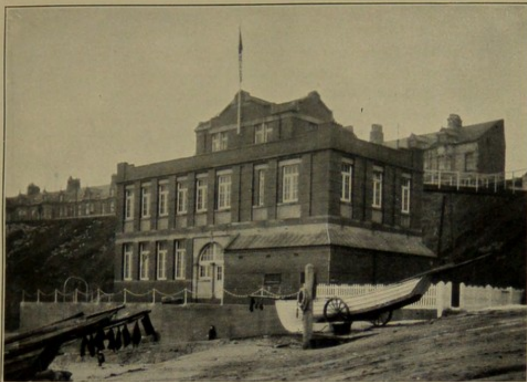
A. GENERAL VIEW, CULLERCOATS, "COBBLE" IN FOREGROUND.
