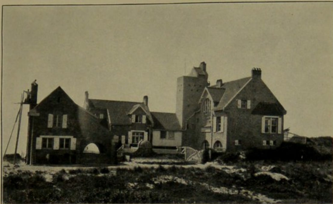
A. STATION BUILDING FROM THE EAST.
