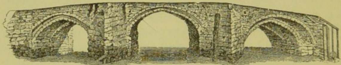
BOW BRIDGE AS IT STOOD BEFORE ITS DEMOLITION IN 1839.
